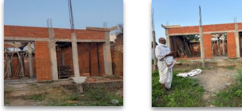
(Left to Right) Image 6 & Image 7: “Building Complex of Vedic Research Institute and Library in memoriam of 42nd and 44th Azhagiyasingars of Ahōbila Mutt and Mukkūr Svāmī” - Under Construction
