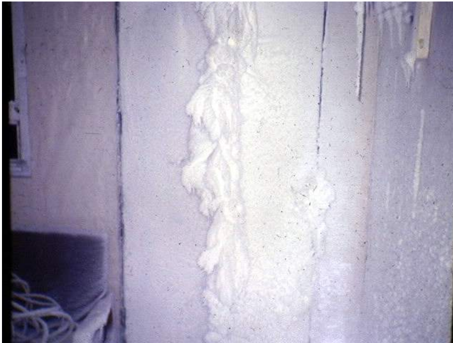
Continuous Blizzard Causes Snow to Turn into Ice Inside Tirumala Doorway
