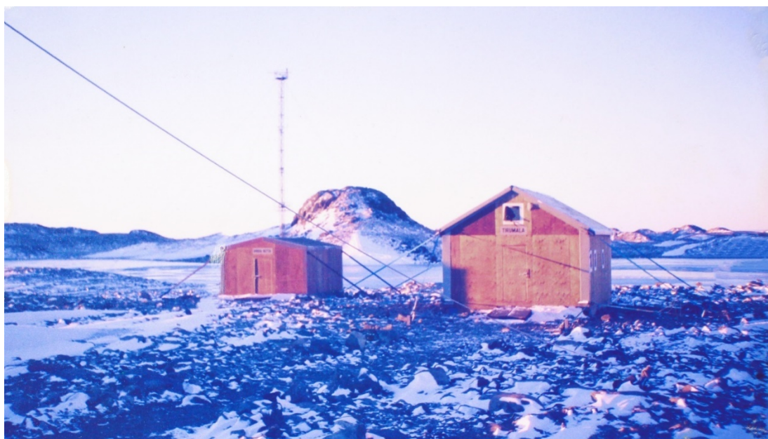
Visible in the image are the effects of overnight snowfall in Schirmacher Oasis, Tirumala, Dodabeta Hut, and a 22-meter mast equipped with wind energy assessment sensors standing tall
