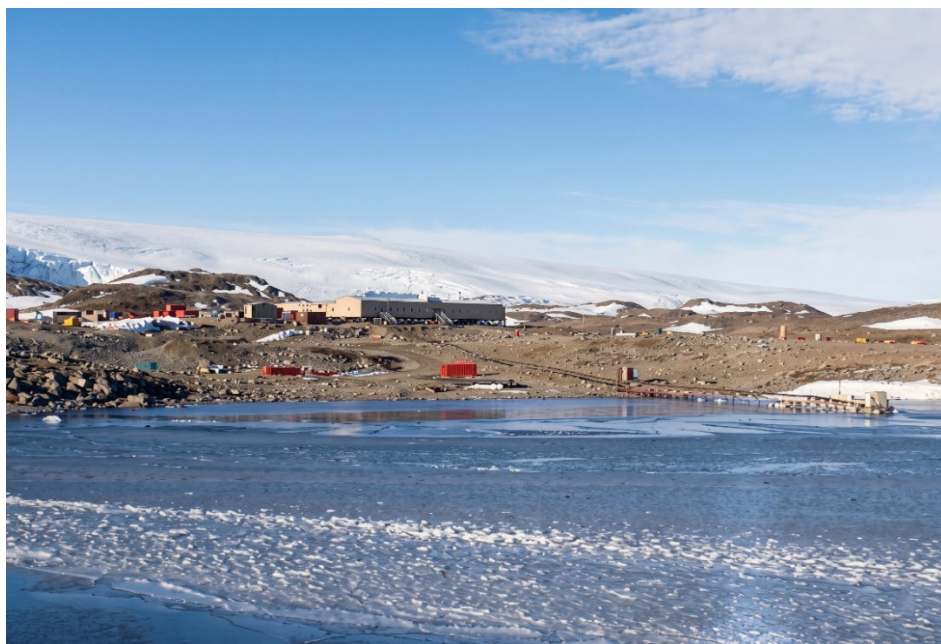
The Pumphouse situated in Priyadarshini Lake, serving as the water source for the Maitri complex
