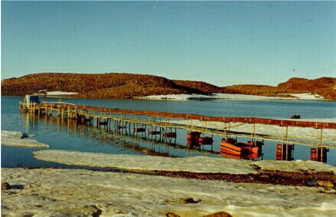
Pipeline conduit carrying water from the pump house to the Maitri complex
