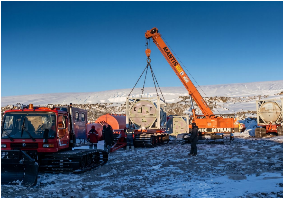
Mantis crane lifting and managing the oil filled tanker brought by convoy team from shelf
