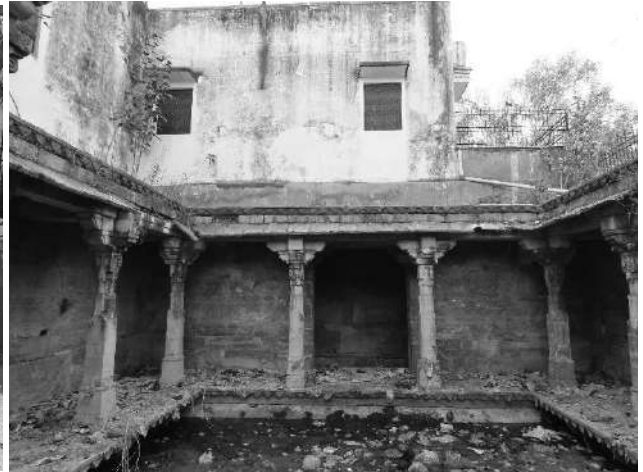
Ghanerao-Jali Vav-pillared corridor on all sides before the well shaft
