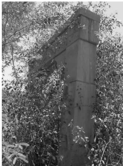
Bhinmal-Pratap Vav-entrance gate
