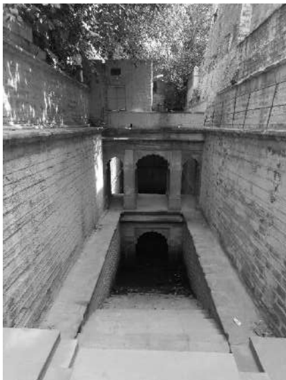
Jodhpur-Nazar ji ki Baodi- showing two storeyed pavilion tower
