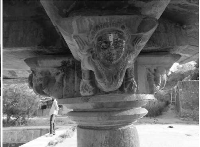
Basantgarh Vav-load bearers in the column capitals of the pavilion
