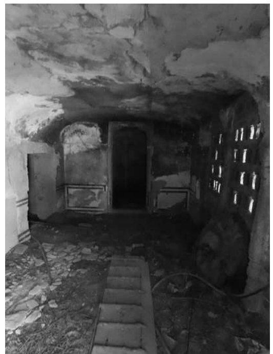
Ramgarh shekhawati-G.B.Ruiya Park Well-chamber with an opening into well shaft
