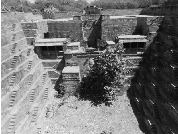
Osian-Katan Baodi -view towards entrance
