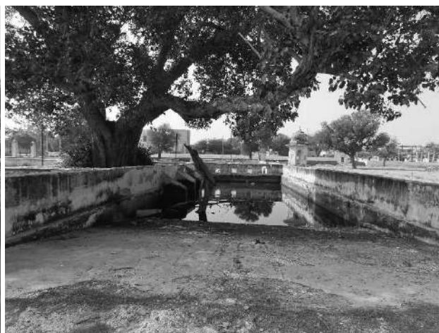
Ramgarh shekhawati-Anantram Poddar ka Johada-ramp for animals with water inlets
