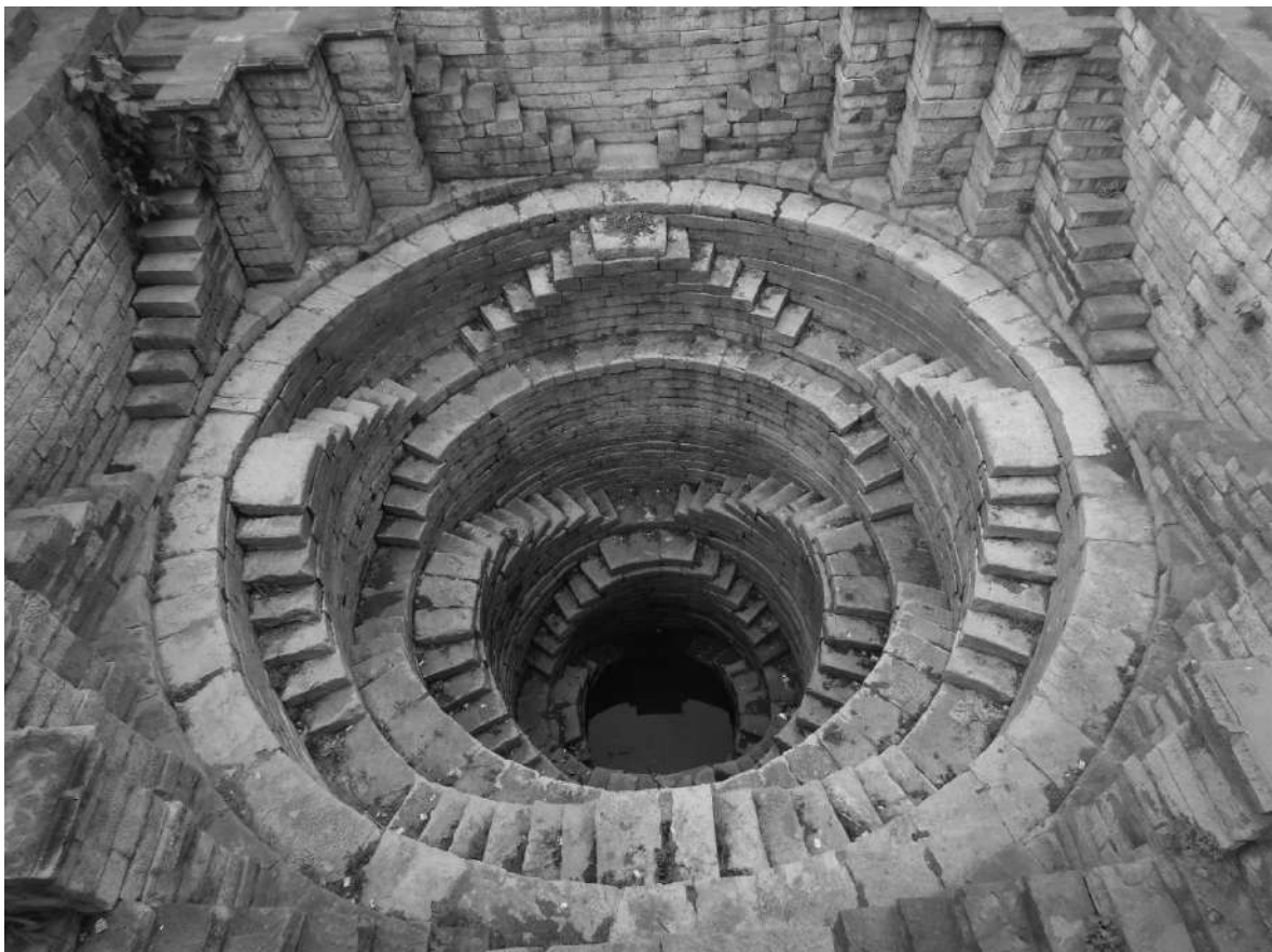
Sukhvas-Kshetrapal Baodi-central vertical well shaft with steps inside
