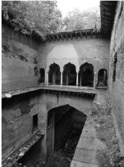
Behror Baodi-second pavilion tower
