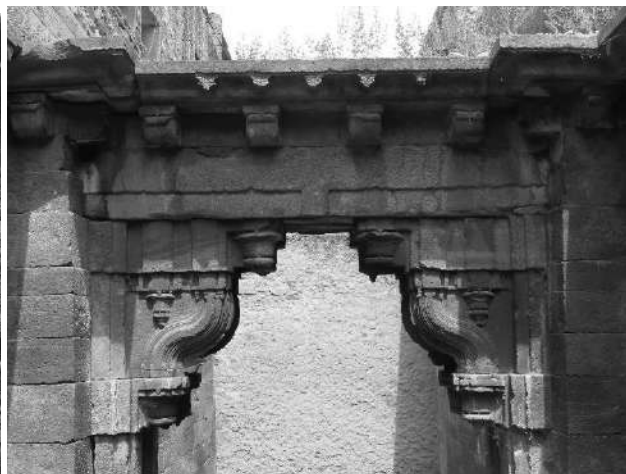
Ransigaon-Bhooton ki Baodi-Corbelled arch of the first pavilion
