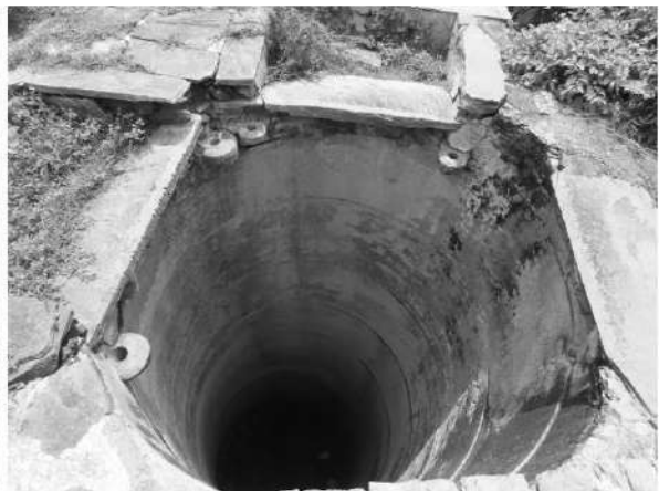
Nayla-Bohron ki Baodi-circular well shaft
