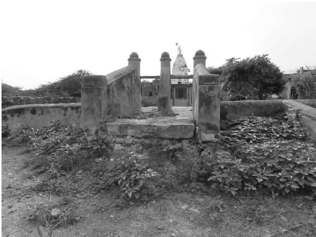
Khandela-Palsaniyon ki Baodi-well shaft
