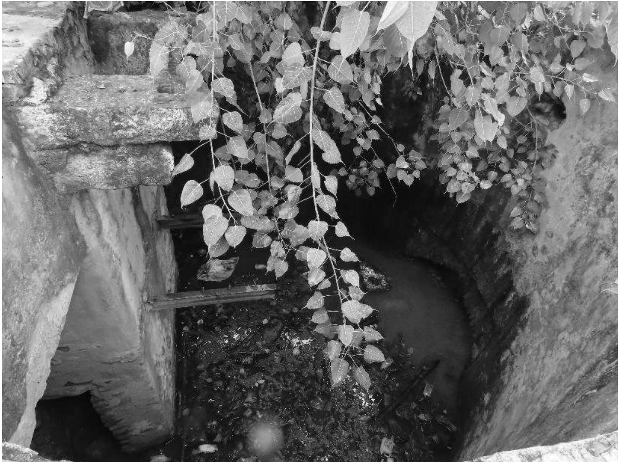
Bahrawanda-Water Works Stepwell-well shaft
