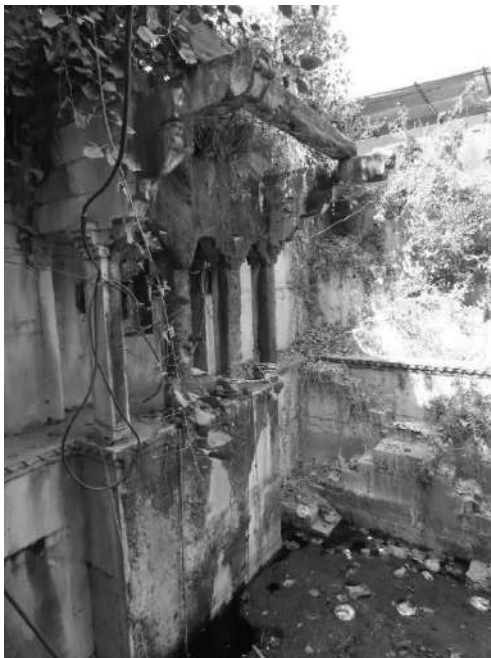
Udaipur-Bedla-Jas Kund- view of the pavilion below the water drawing platform on the north wall
