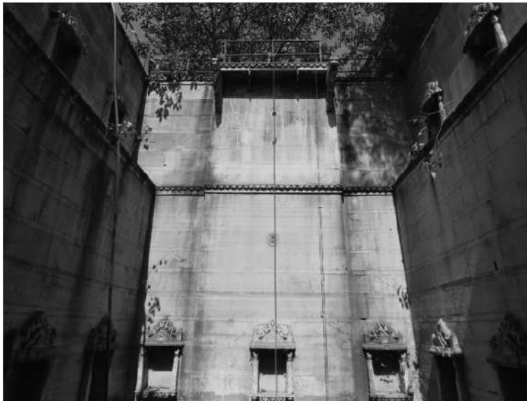
Udaipur-Rajrajeshwar Mahadev Baodi-view towards the well shaft
