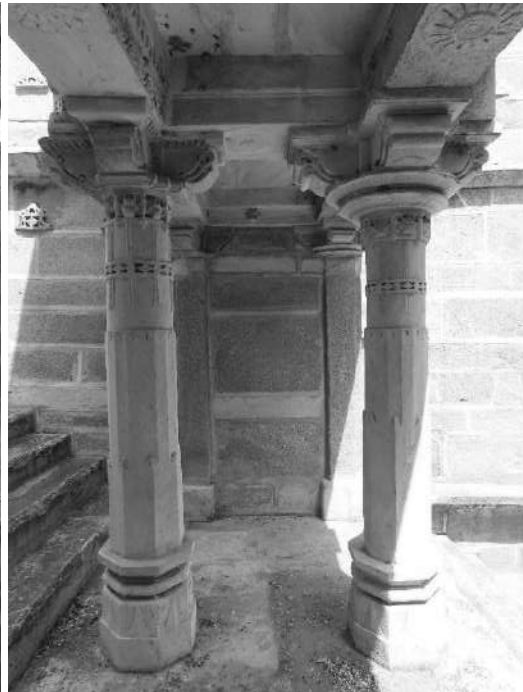
Nadol-Ashapura Mataji temple stepwell-carved columns
