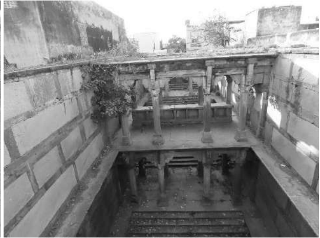
Salemabad-Chor Baodi-second pavilion tower from well shaft side
