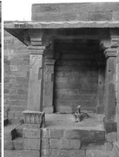
Sukhvas-Kshetrapal Baodi-corner chhatri supported on four columns
