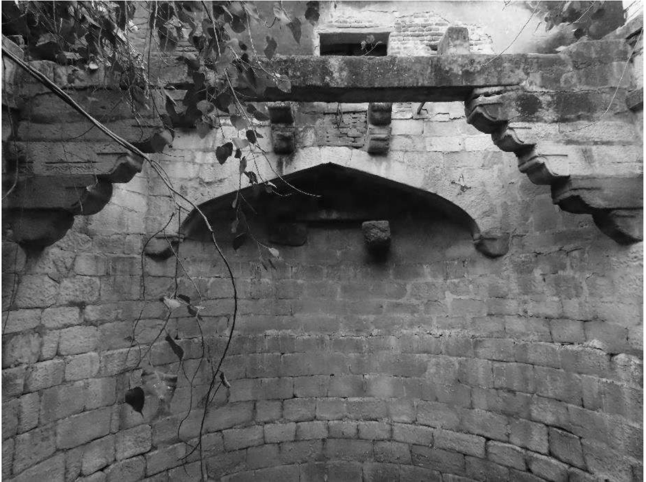
Ghanerao-Mailli Vav-circular well shaft showing water drawing arrangement
