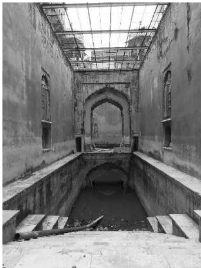
Bundi-Bhawalde ki Baodi-two storeyed second pavilion tower
