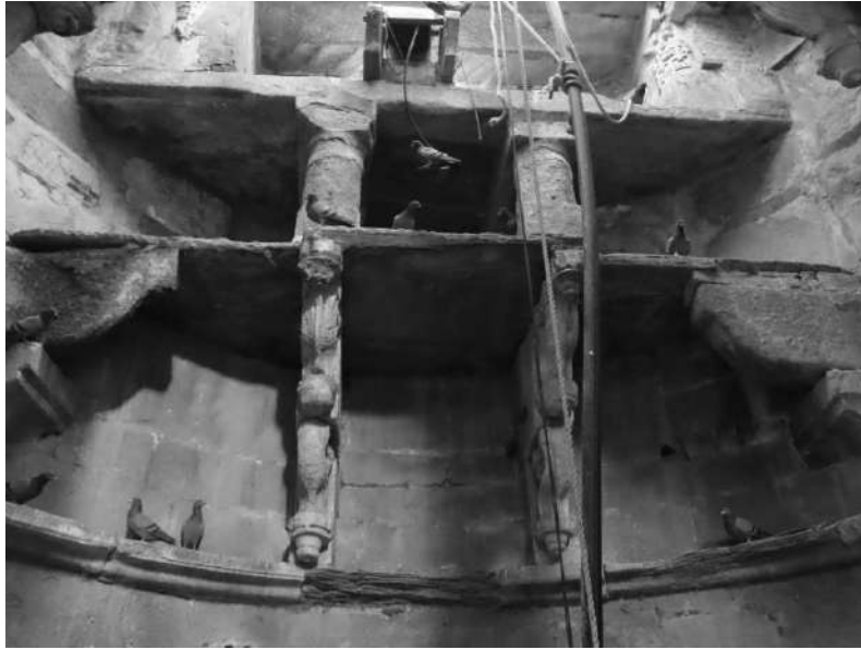
Sadri-Tarachand Kavedia Baodi-water drawing arrangement on top of the well shaft
