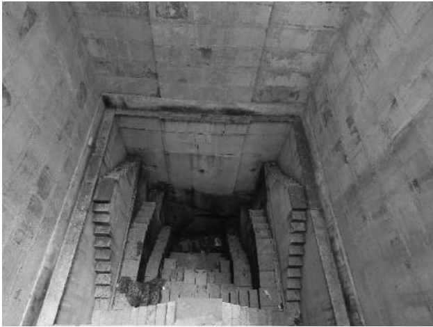
Bundi-Nahar Dhoos ki Baodi- looking down the well shaft
