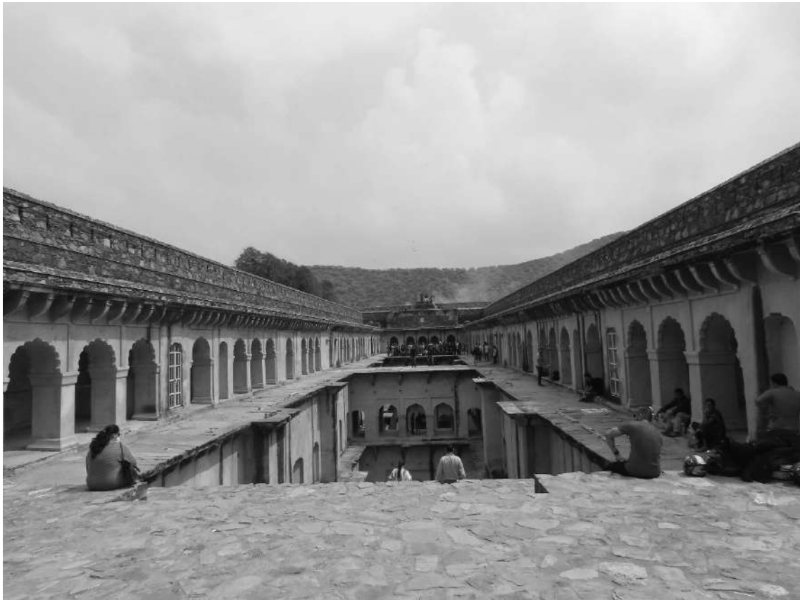
Neemrana Baodi- view at the ground level from the entrance
