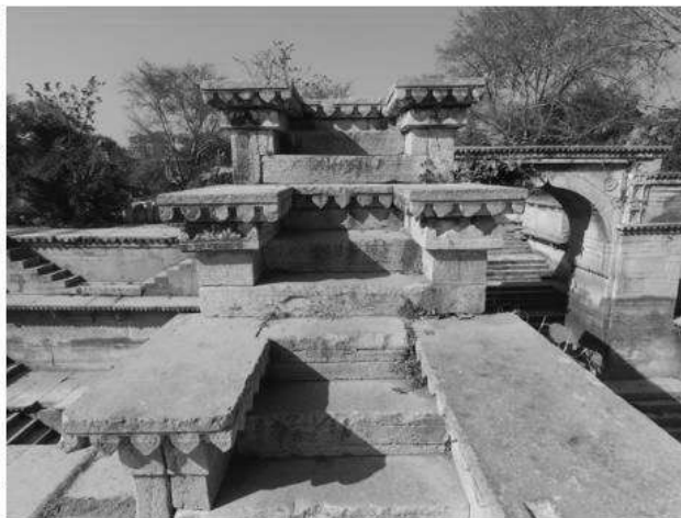
Binota ki Baodi-steps to go to the top of the entrance pavilion tower
