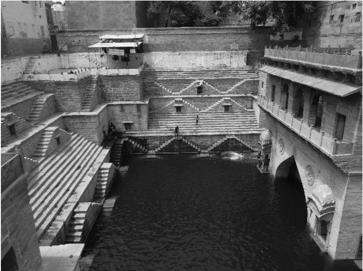
Jodhpur-Toor ji ka Jhalra-another view showing unauthorised structure
