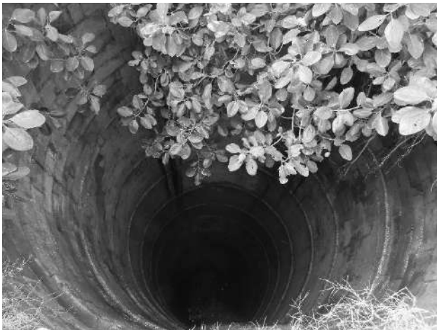
Machadi-Bairwa Basti Boadi-circular well shaft
