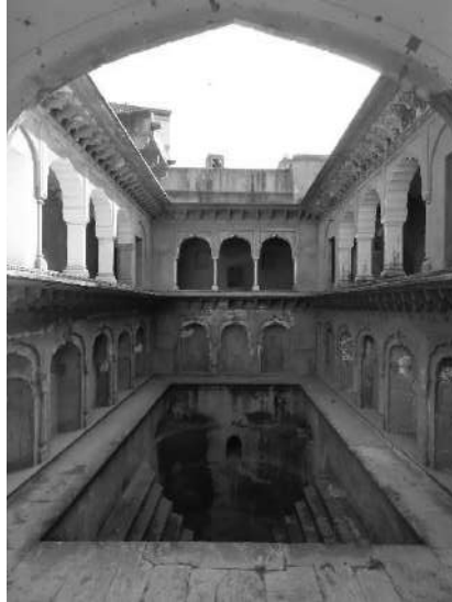
Shahpura Baodi-view from the first tower
