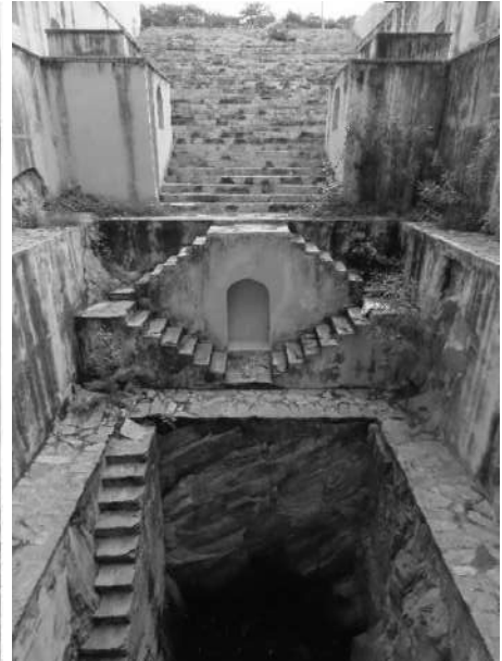
Jaipur-Amber-Maaji ki Baodi-view towards the entrance in the west
