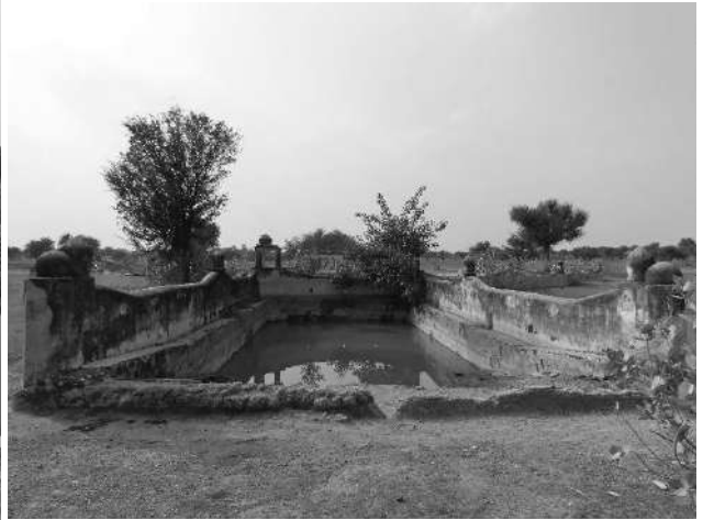
Untwaliya ka Johada-ramp for animals and inlet for water
