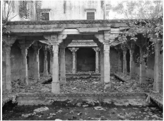
Ghanerao-Jali Vav-view of the second pavilion tower
