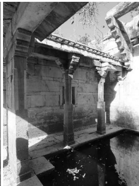
Ghanerao-Brahmapuri Baodi-showing water drawing arrangement in the east and one of the two side pavilions below it
