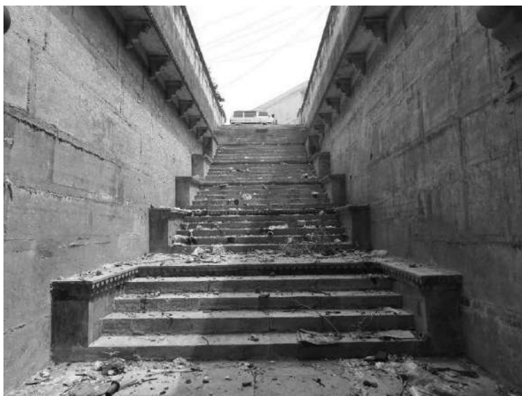
Pench ki Baodi-Ganesh ji ki Baodi-view of the entrance from the south
