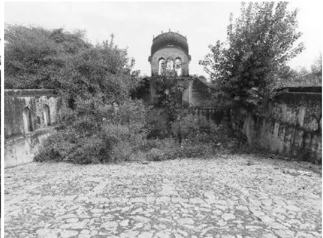
Lakshmanagarh-Bhadrana Johada-ramp for animals and water inlet to Johara
