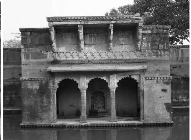
Gendoli-Bada Kund-pavilion and water hauling arrangement in the south
