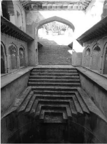
Shahpura Baodi-view from the well shaft
