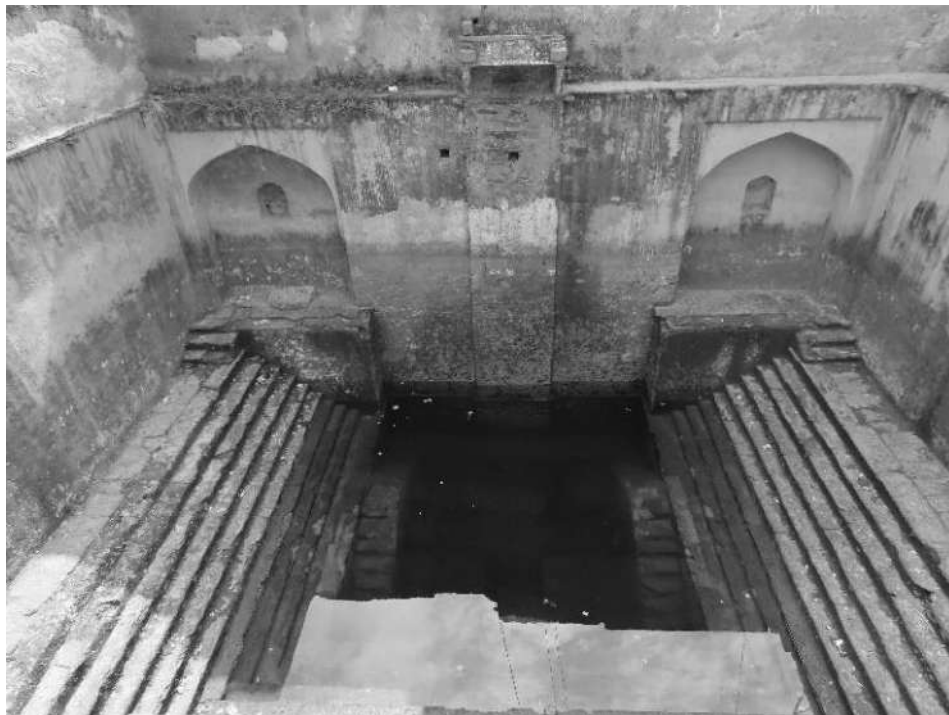
Sawai Madhopur -Thathera Kund- view from the western entrance
