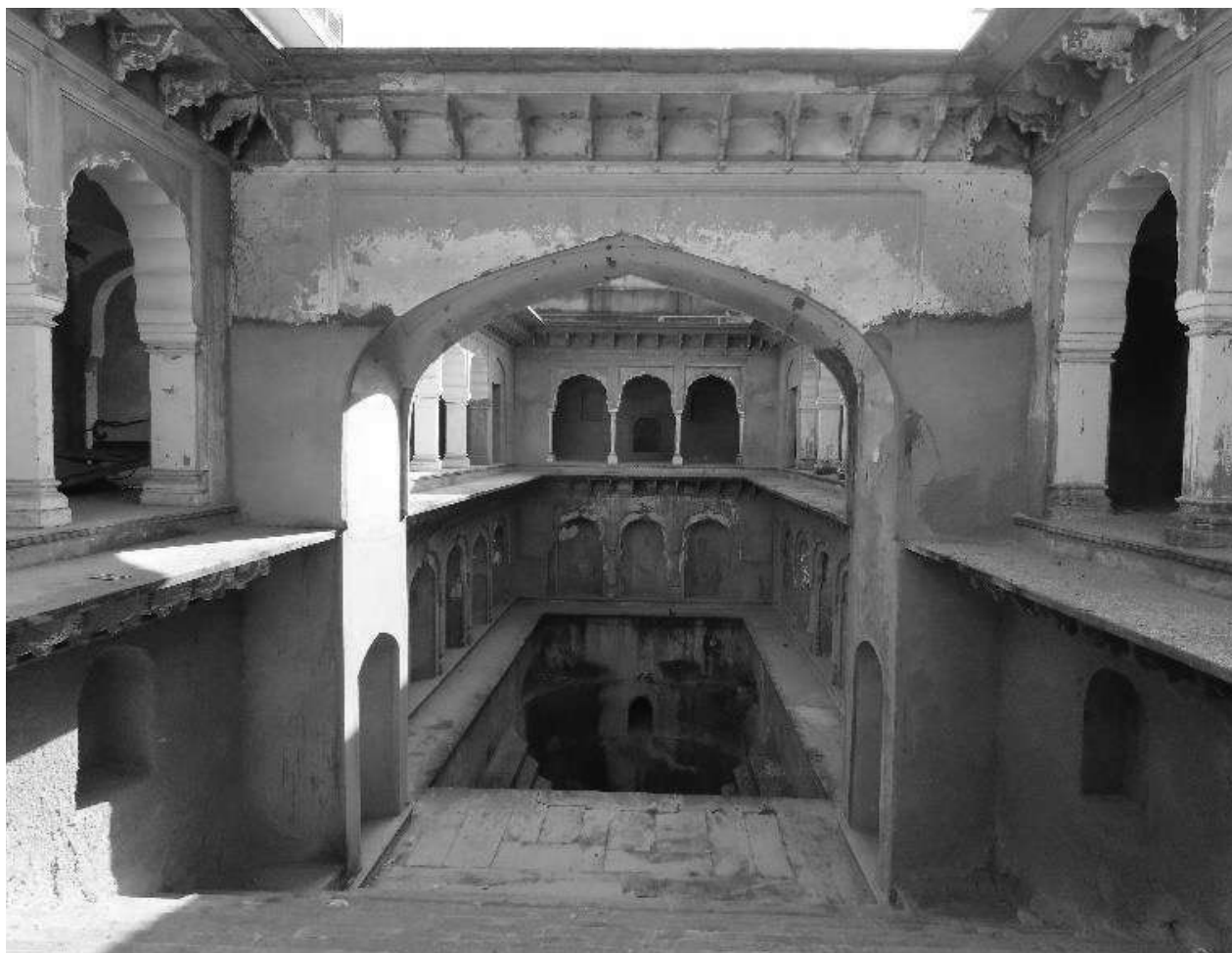
Shahpura Baodi-first pavilion tower in the foreground
