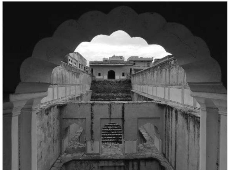
Jaipur-Amber-Gangadas ki Baodi -view through the multifoil arch opening of the top pavilion
