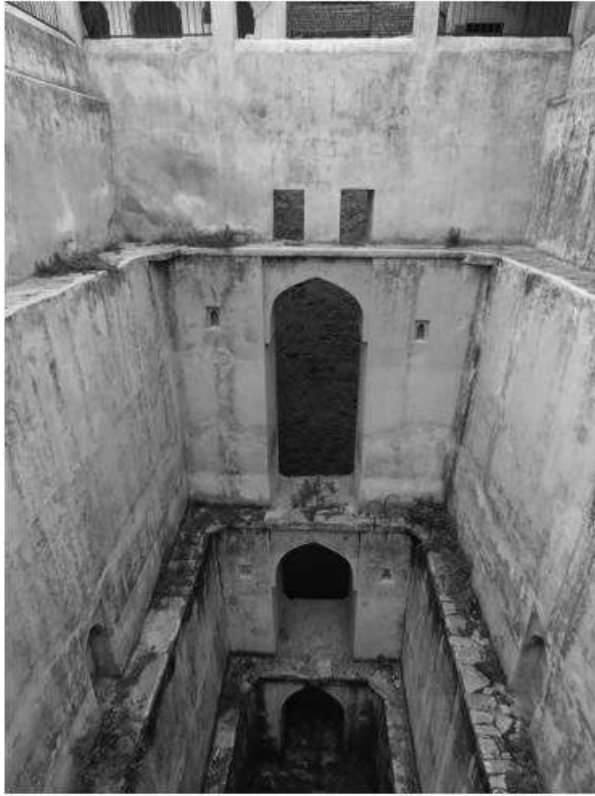
Jaipur-Amber-Naku ki Baodi-view of the third half pavilion tower connected with well shaft
