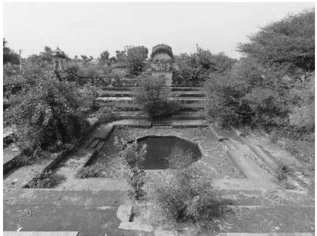
Lakshmangarh-Bhadrana Johada-vegetation growth inside johada
