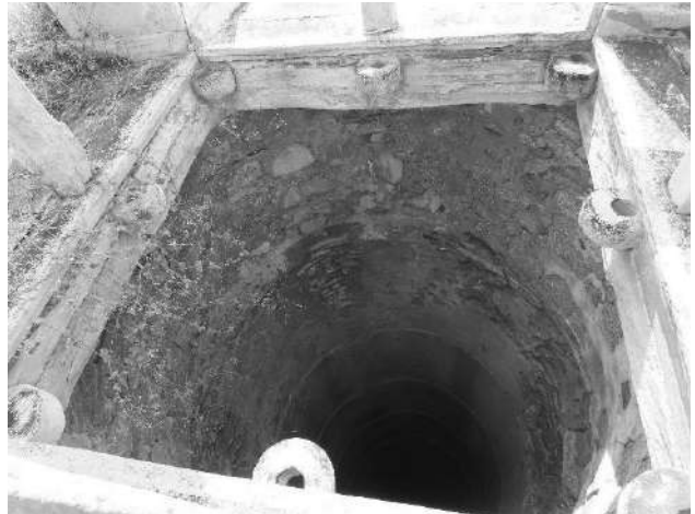
Lakshmangarh-Bhadrana Kua-well shaft with water hauling arrangements
