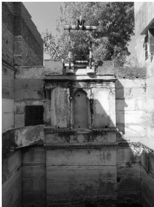
Bhinder-Hijron ki Baodi-well shaft and water fetching arrangement in the west
