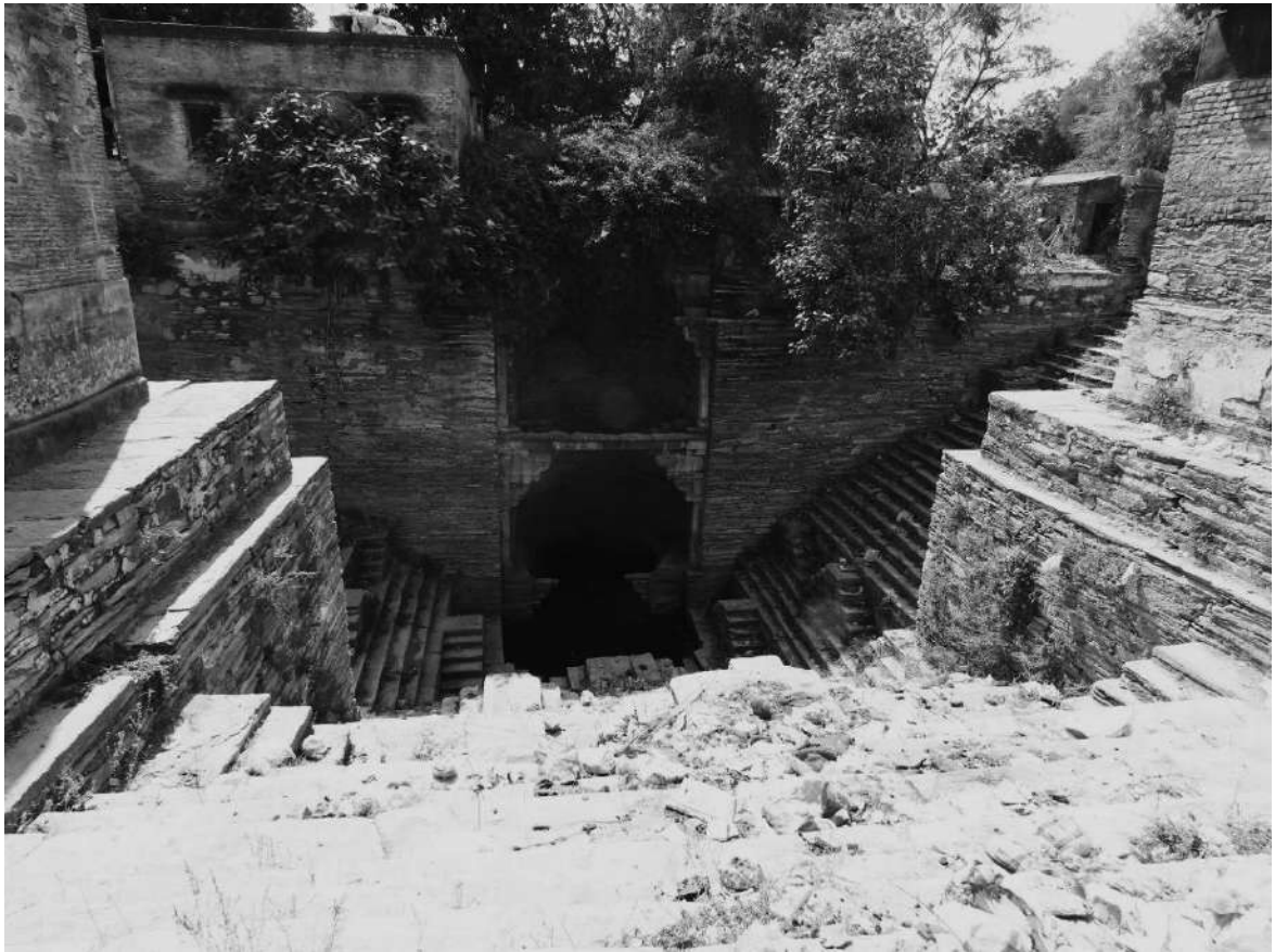
Sirohi-Champawati-Ram Jharokha Mandir Baodi- View towards the well shaft
