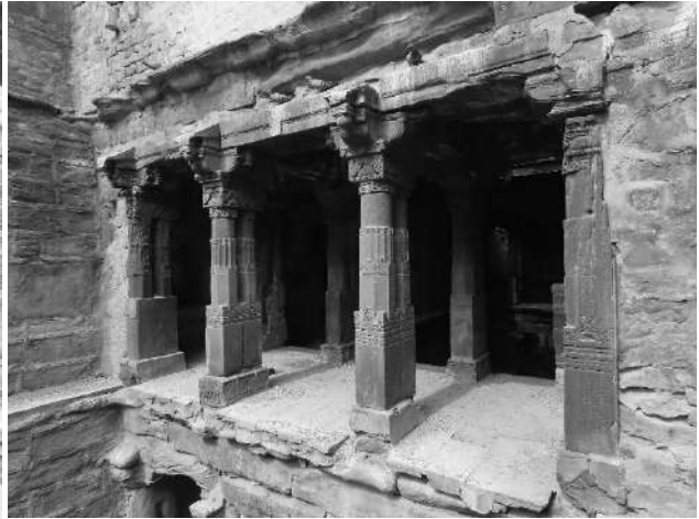
Jodhpur-Tapi Baodi-another type of columns having various cross sections
