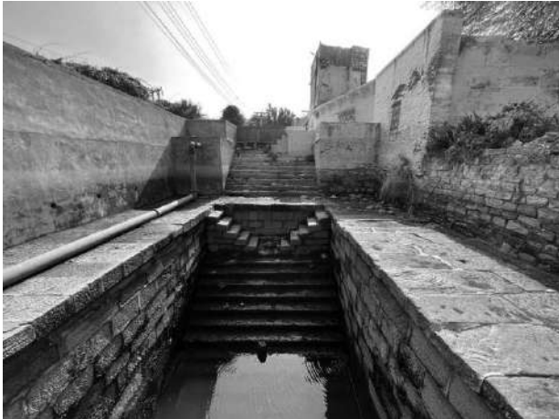
Jodhpur-Kharbuja Baodi-as viewed from the north end
