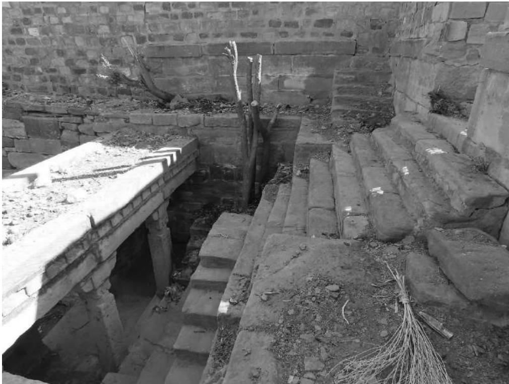
Baodi at Baori-showing the steps coming down from the entrance and the only pavilion below it
