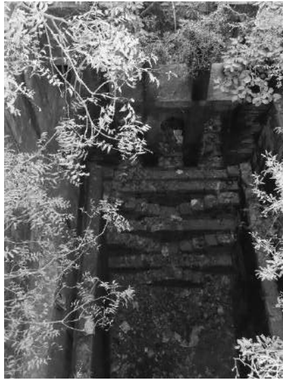
Khandela-Kali Bai ki Baodi-steps in the auxiliary tank
