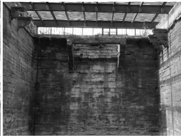
Jodhpur-Eidgah Baodi- well shaft with water drawing arrangement
