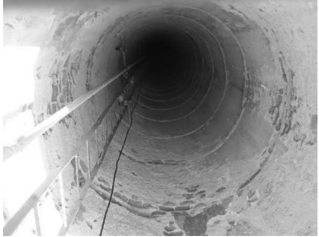
Fatehpur Shekhawati-Poddaron ka Kua-well shaft
