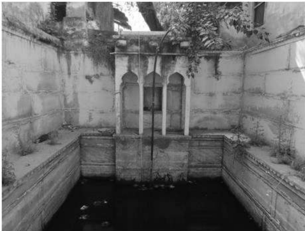
Bhinder-Baiji Raj ki Baodi-view of the well shaft and water drawing arrangement in the south
