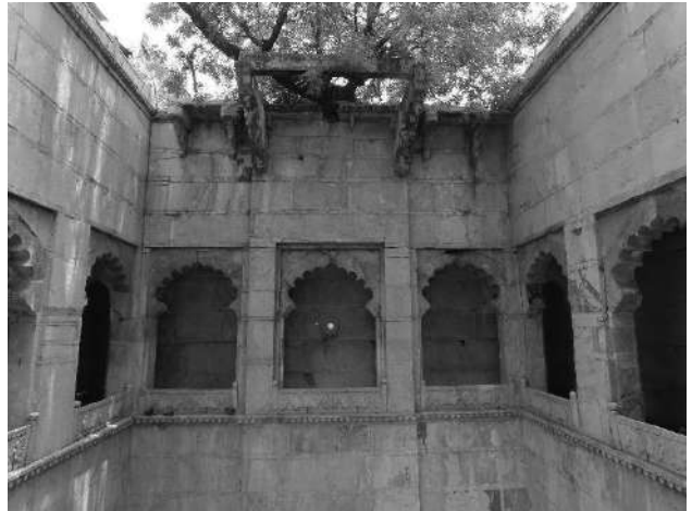
Bundi-Nahar Dhoos ki Baodi-verandahs around the well shaft
