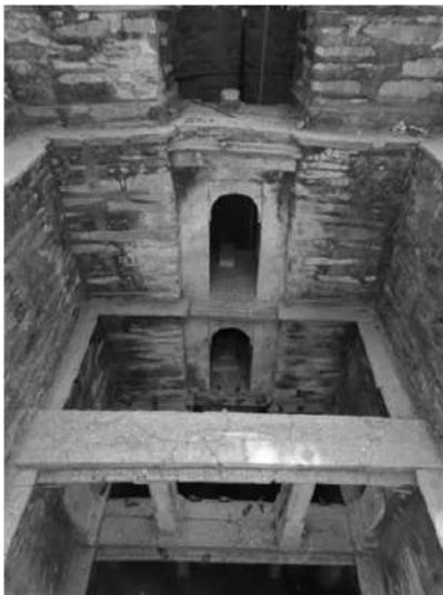
Sirohi-Sarja ki Baodi-view of the last ardh-koot and the openings in the well shaft connecting the stepped corridor
