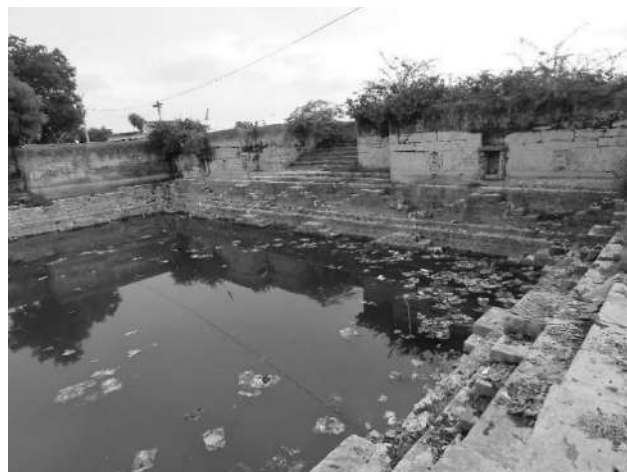
Lakheri-Jind Baba ka Kund-showing niches and entrance steps
