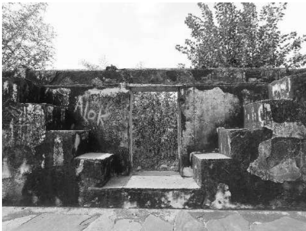
Lakshmanagarh-Bhadrana Johada-another type of water inlet and entrance to Johad
