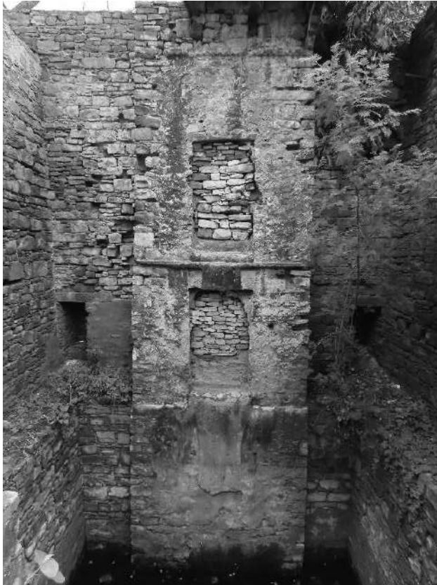
Chhan ki Baodi-well shaft
