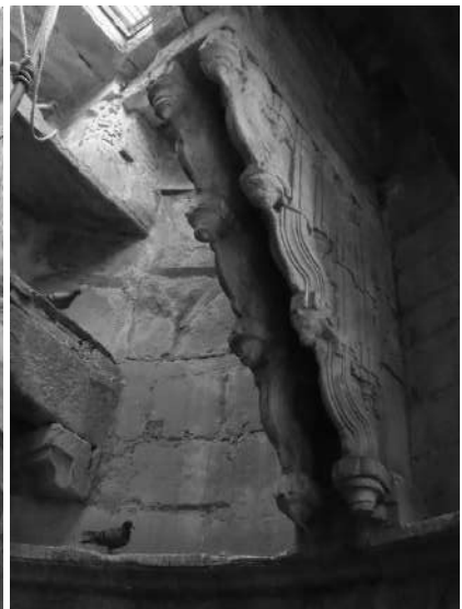
Sadri-Tarachand Kavedia Baodi- carved bracket of water drawing arrangement
