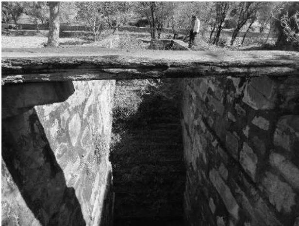
Sakat-Baba Khaqnath ki Baodi-view from the well shaft towards entrance
