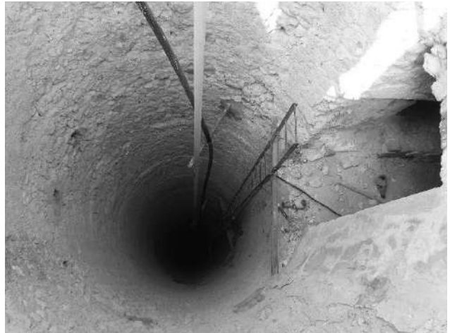
Ramgarh shekhawati-G.B.Ruiya Park Well-well shaft with an opening
