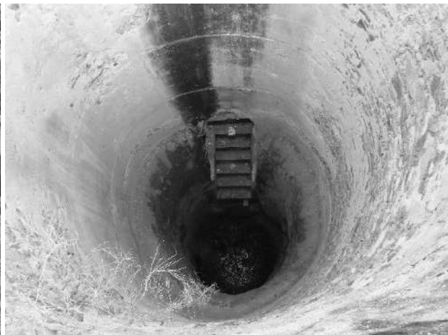
Marwa Baodi-view of well shaft from the top showing connection with the corridor
