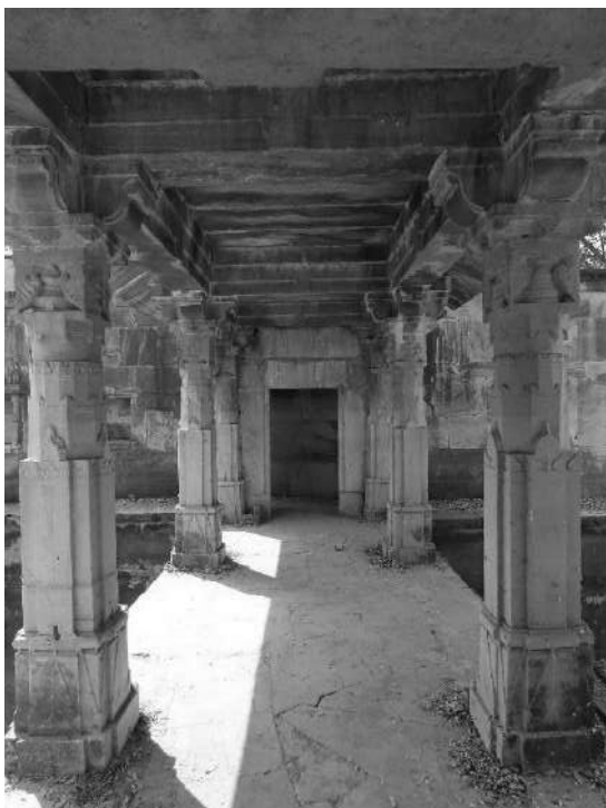
Udaipur-Sundarbhai ki Vav- view of top pavilion of the second pavilion tower
