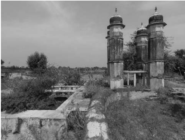
Lakshmangarh-Bhadrana Kua-showing the ramp for driving bullocks
