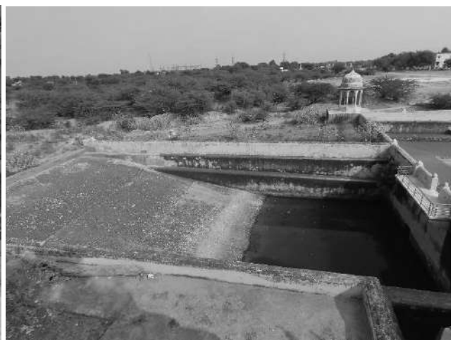
Bissau ka Johada-ramp for animals and inlet for water
