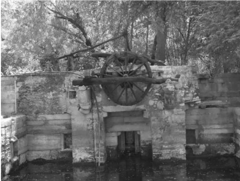
Narlai-Amba Vav-rehat in the south of the stepwell
