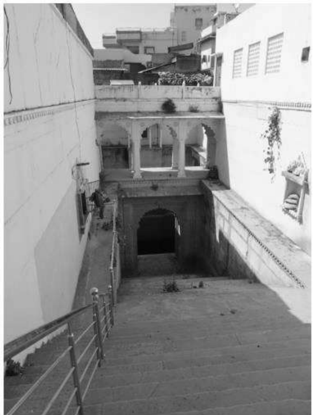
Badi Sadri-Charbhuja Kharagli Baodi-view from the entrance
