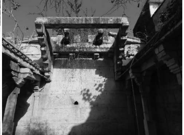
Ghanerao-Brahmapuri Baodi-water drawing arrangement in the east
