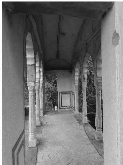
Lakshmangarh-Todi College Johara-inside view of a pavilion
