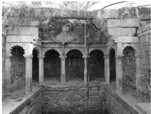
Ghanerao-Dungaria Baodi-galleries surrounding the well shaft
