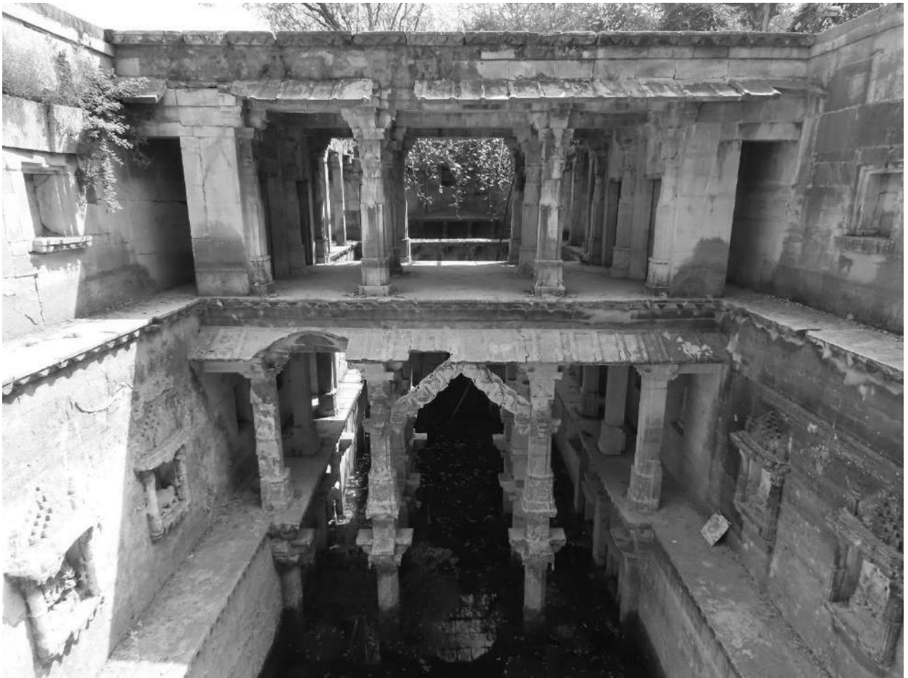
Udaipur-Sundarbai ki Vav- view of the third pavilion tower with toran openings in the lower storey
