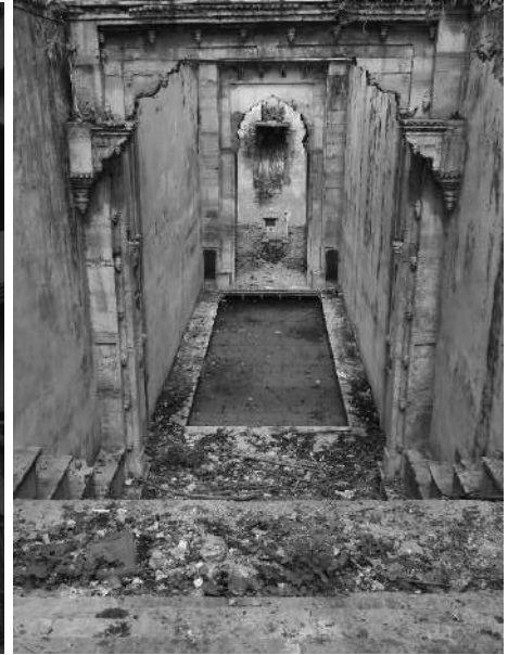
Bundi-Naruki Baodi-showing first pavilion with corbelled arch and kund before the second pavilion tower
