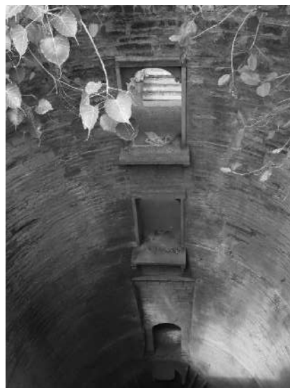
Manch-Jind Baba ki Baodi -well shaft
