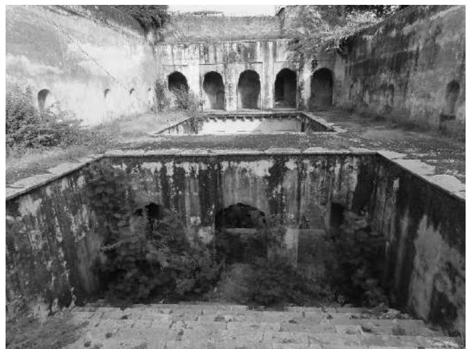
Khandela-Munka ki baodi-view of the two pavilion towers
