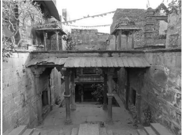
Balunda Stepwell-first pavilion tower
