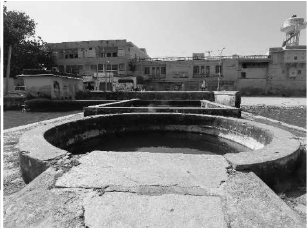
Naraina-Gaurishankar Baodi-view from the well shaft
