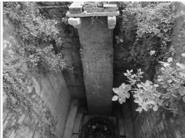
Sawai Madhopur-Alanpur baodi-well shaft in the east
