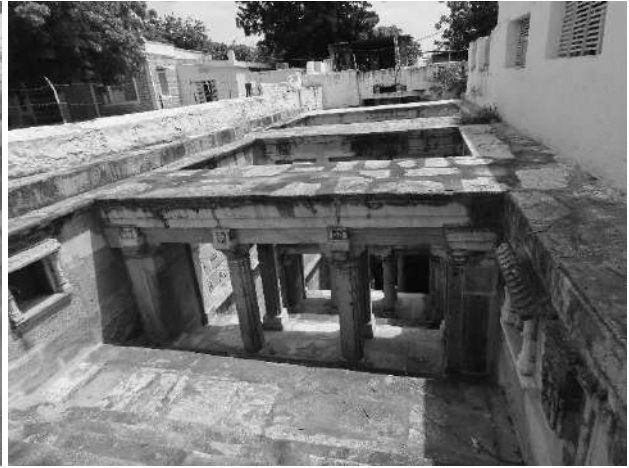
Nadol-Ashapura Mataji temple stepwell-view of the stepwell from the entrance with first pavilion tower in the foreground
