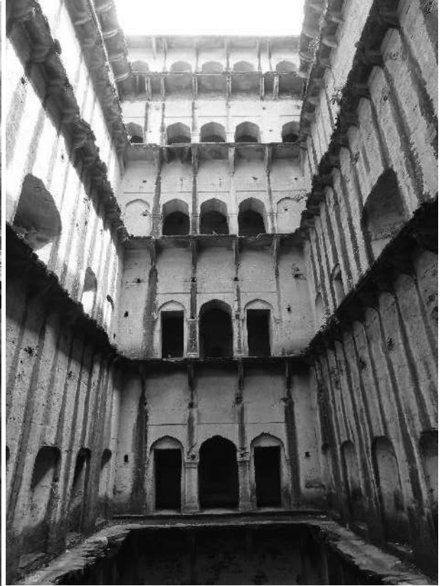
Neemrana Baodi-upper storeys of third pavilion tower
