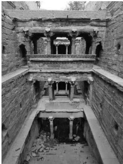
Jodhpur-Tapi Baodi-third pavilion tower
