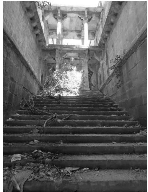
Lavera Kalan stepwell-second pavilion tower when seen towards entrance
