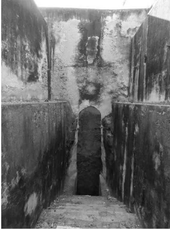
Marwa Baodi-showing connection between well shaft and stepped corridor
