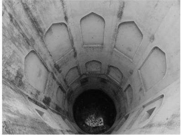
Jaipur-Amber-Rukmani Baodi- looking down the well shaft
