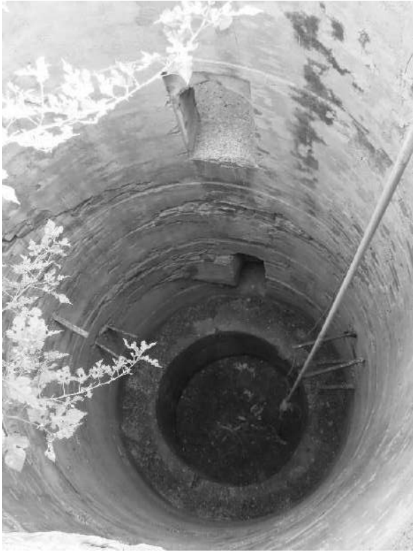
Todalari ki Baodi-well shaft with openings to connect the stepped corridor
