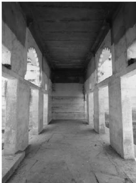
Badi Sadri-Charbhujia mandir Baodi- upper storey of the pavilion tower
