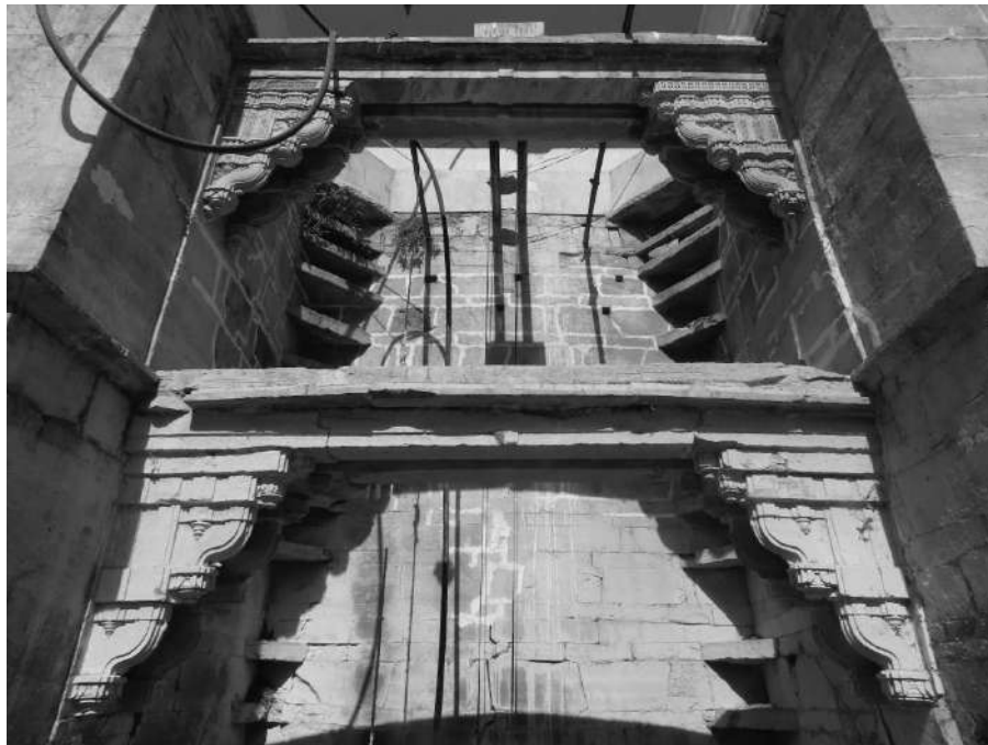
Sirohi-Ratan Baodi -water drawing arrangement at the well shaft with brackets
