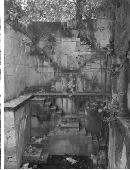
Udaipur-Bedla-Jas Kund- view of the south wall with descending steps
