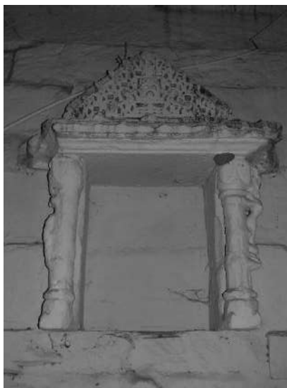
Sewari-Jaital Vav-another niche in the side wall
