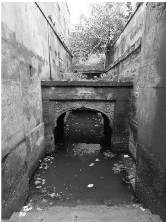
Jodhpur-Chand Baodi-showing a pointed arch pavilion
