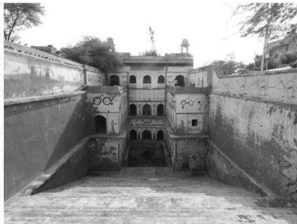
Dausa-Banidas ki Baodi-view towards the pavilion tower
