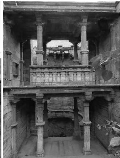
Balunda Stepwell-second pavilion tower with the well shaft in the background
