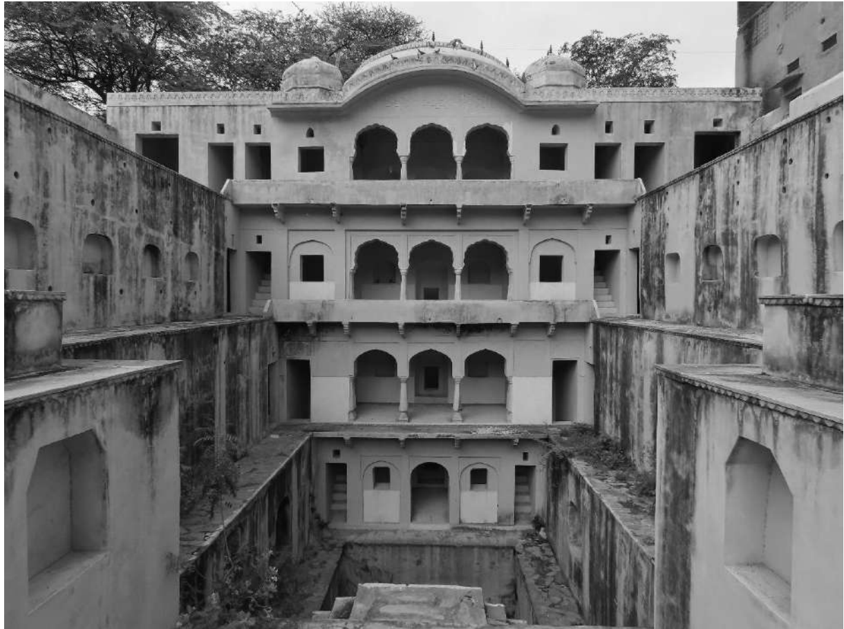
Jaipur-Amber-Maaji ki Baodi-four storeyed pavilion tower in the east
