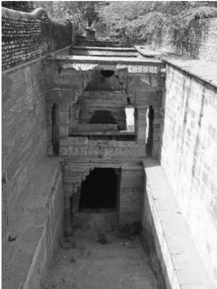
Rajlani baodi-view from the top of the first pavilion tower
