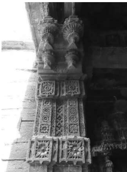
Rajlani baodi-twin-pillared column of the first pavilion on right hand side
