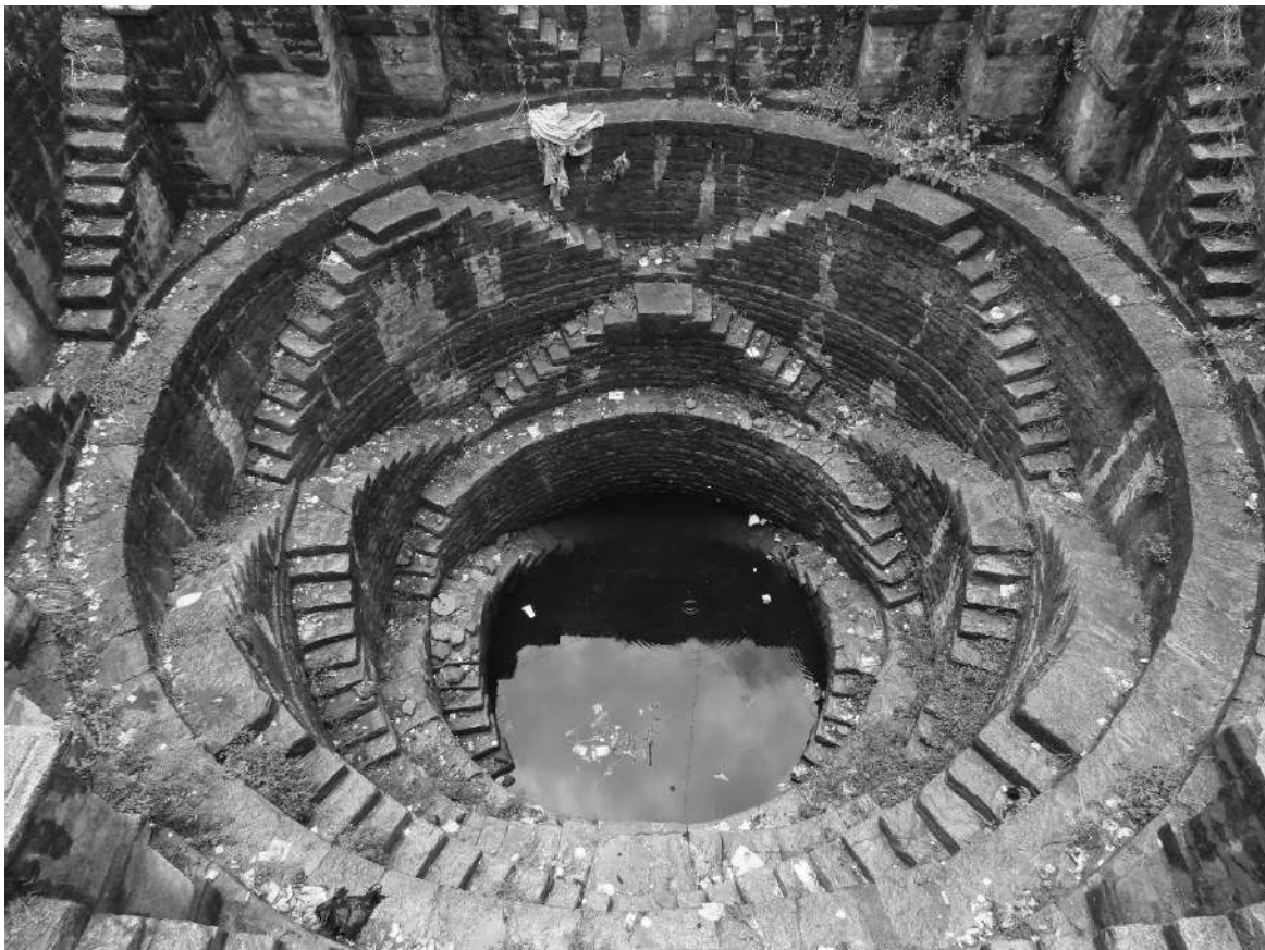
Allapur Baodi-circular well shaft with steps inside
