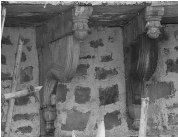
Machadi-Rani ka Kua-beautiful corbels at the first level
