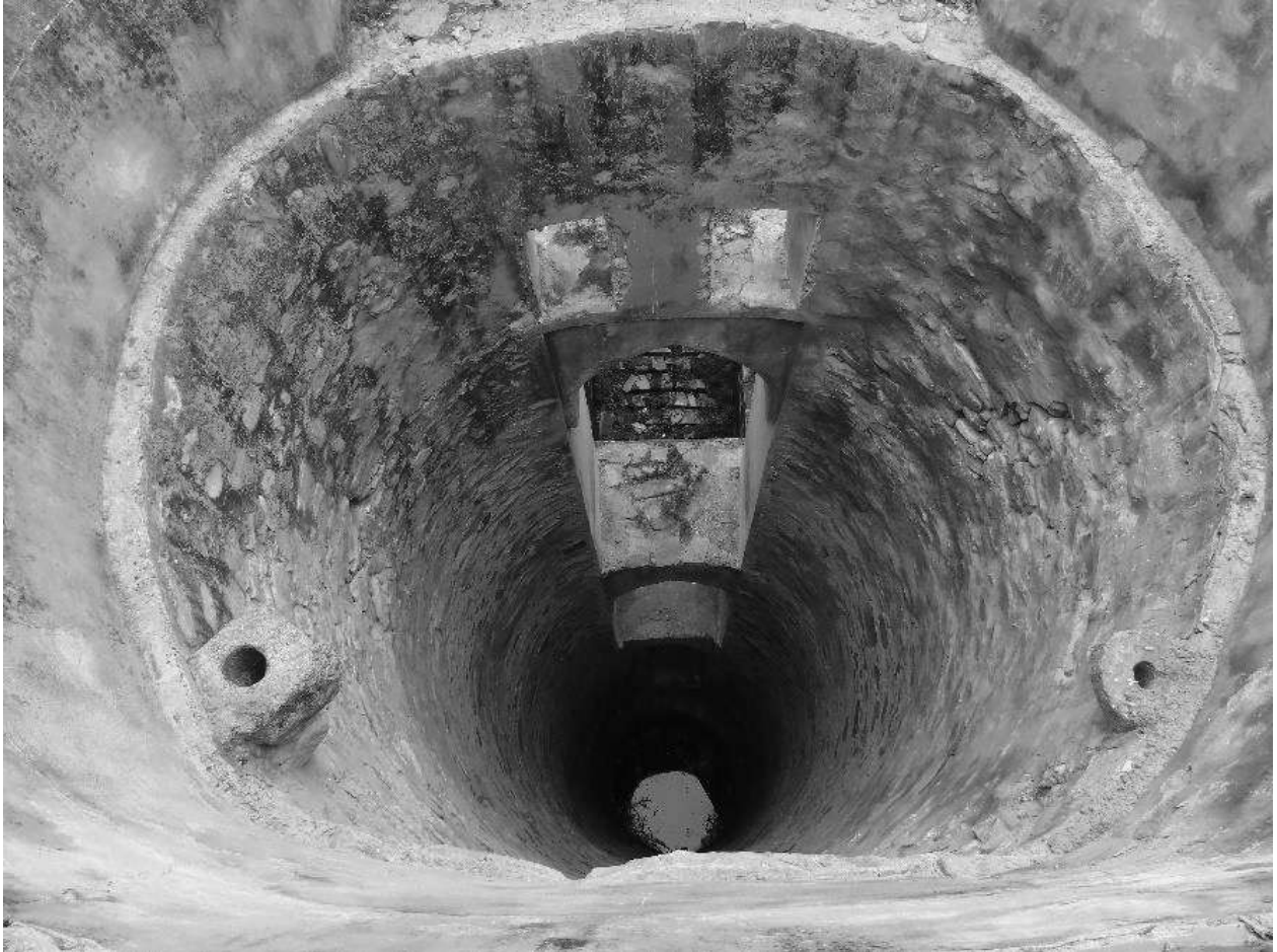
Jaipur-Amber-Naku ki Baodi-circular well shaft with openings into stepped corridor
