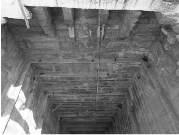
Nadol-Ashapura Mataji temple stepwell- well shaft
