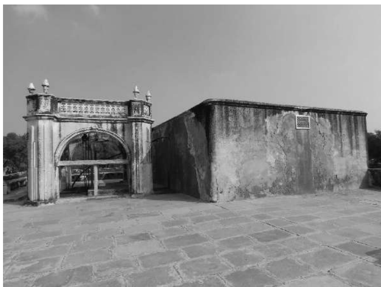
Ramgarh Shekhawati-G.B.Ruiya Jalashaya-pillars for supporting water lifting arrangement and storage tank
