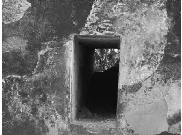
Lakshmangarh-Bhadrana Johada-water inlet from the ramp outside Johada
