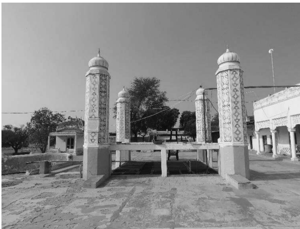
Fatehpur Shekhawati-Pinjrapole Society Kua-pillars around the well shaft
