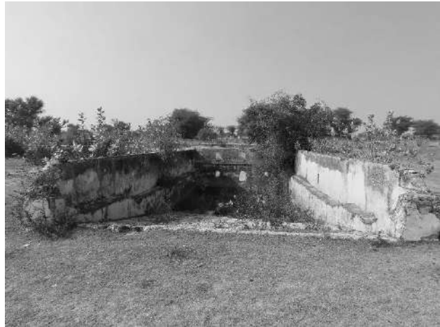
Rolsabsar Johadi-ramp with water inlets
