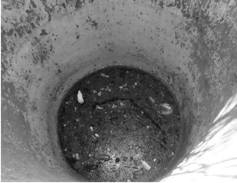
Tehla- Laseda Baodi-circular well shaft
