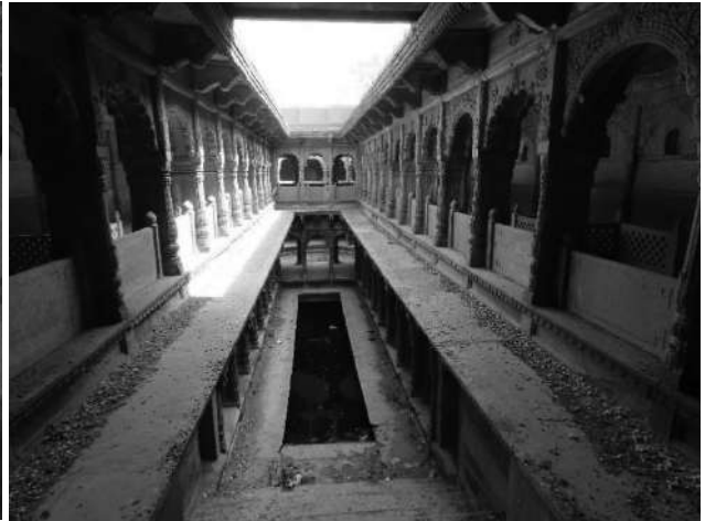
Dhaulpur-Chhoti Baodi- view of top storey
