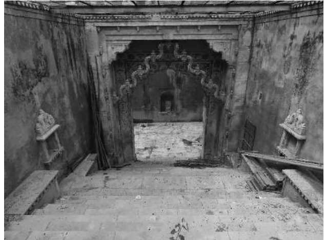
Bundi-Bhawalde ki Baodi-toran gate of the first pavilion
