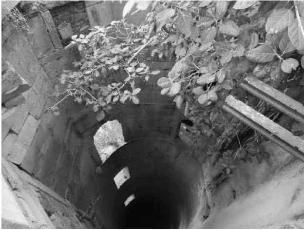
Khandela-Songiri Baodi-looking down the well shaft
