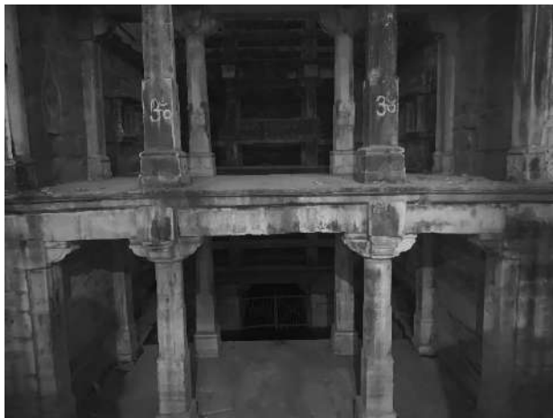
Sewari-Jaital Vav-lower two storeys of the third pavilion tower
