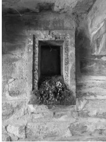
Baodi at Baori- the niche in the pavilion
