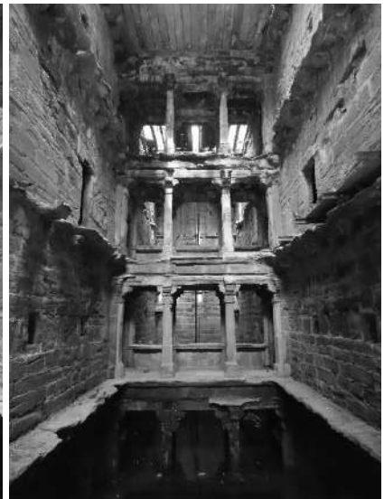
Jodhpur-Tapi Baodi-five storeyed pavilion tower
