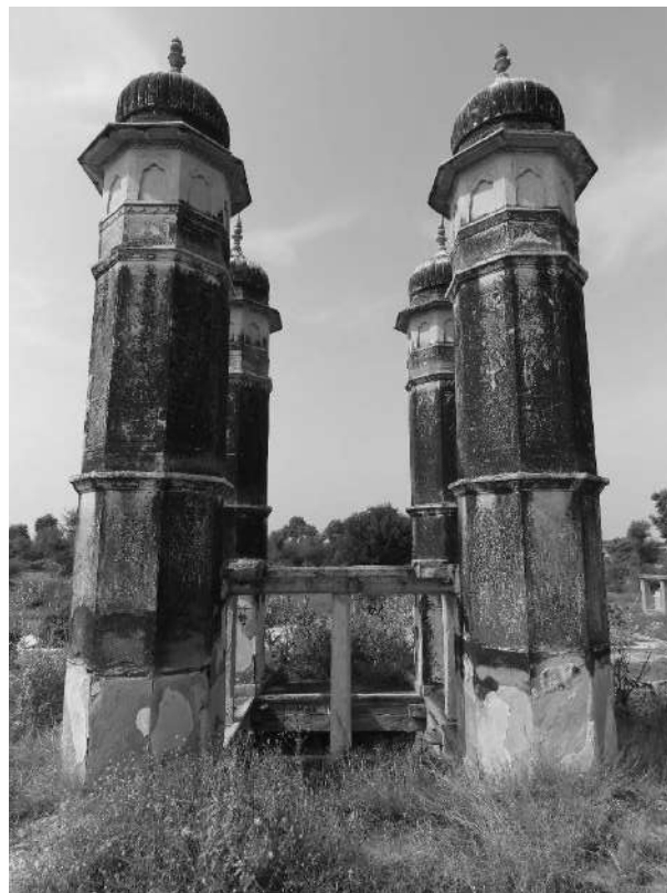
Lakshmangarh-Bhadrana Kua-pillars are supporting the water hauling arrangement
