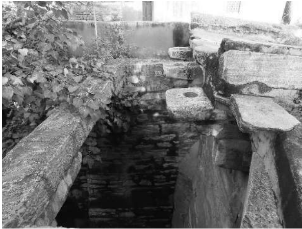
Kotputli-Nagaji ki Baodi- water drawing platform
