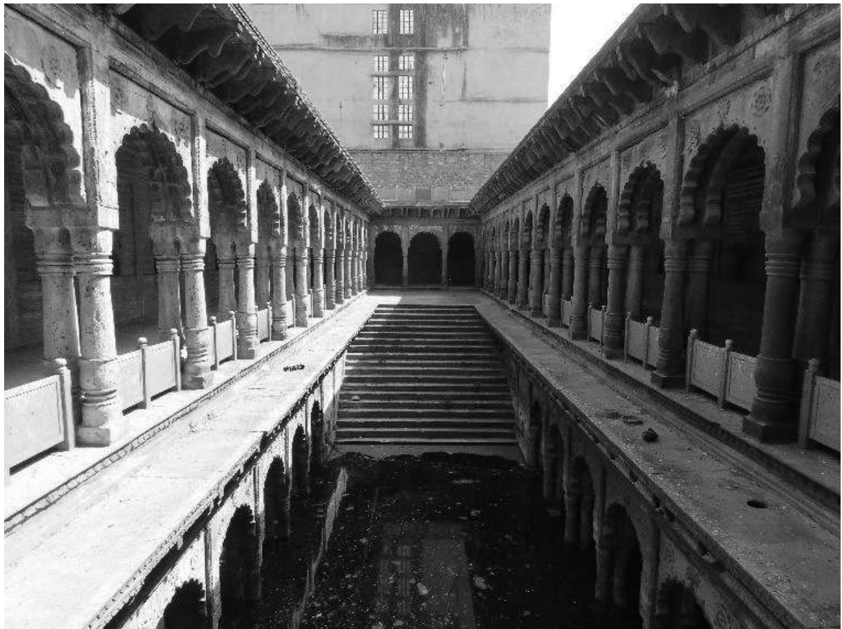
Dhaulpur-Royal stepwell-view of the stepped corridor with side pavilions from the west
