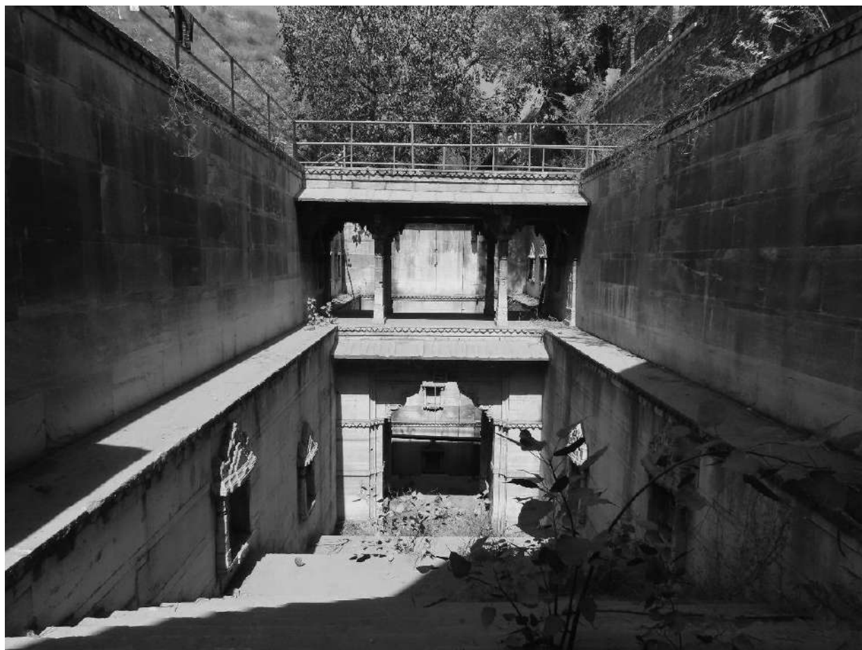
Udaipur-Rajrajeshwar Mahadev Baodi-view of the second pavilion tower
