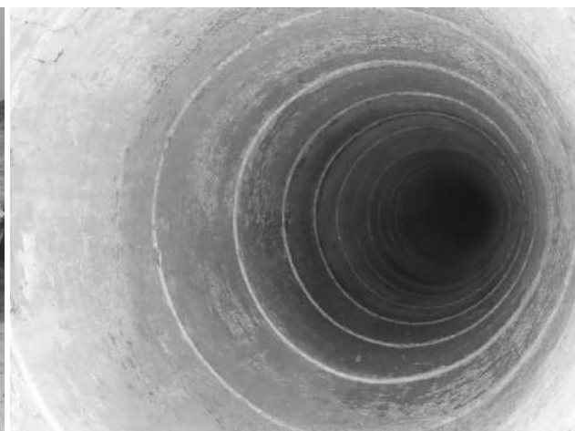
Lakshmangarh-Dholas ka Kua-well shaft
