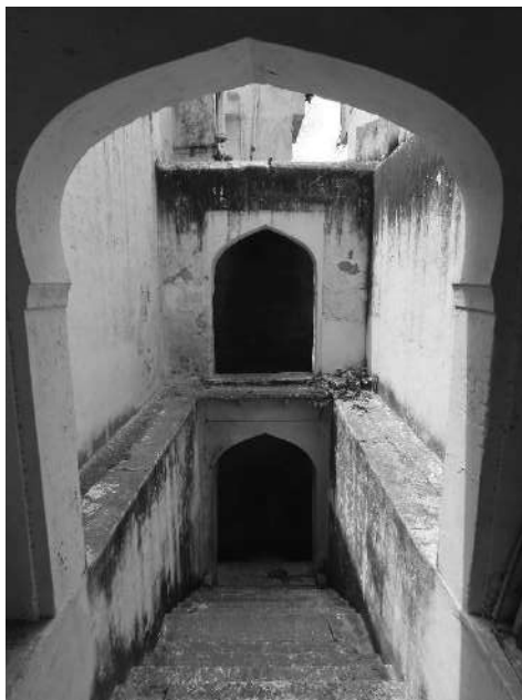
Sawai Madhopur -Thathera Kund- view from the western entrance
