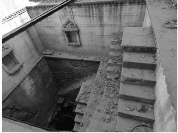
Udaipur-Rajrajeshwar Mahadev Baodi-steps in the well shaft
