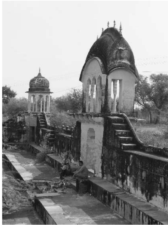
Lakshmanagarh-Bhadrana Johada-steps connecting the pavilion and central entrance in the middle and chhatra at the corner
