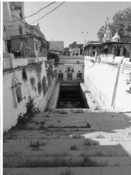
Badi Sadri-Charbhujia mandir Baodi-East- west orientation of the stepwell as viewed from the entrance
