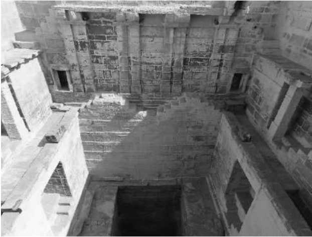
Sathin-Bheru ji ki Baodi-view of the stepped well shaft from the tower
