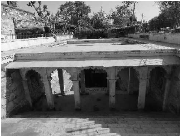
Ghanerao-Dungaria Baodi-first pavilion tower in the foreground
