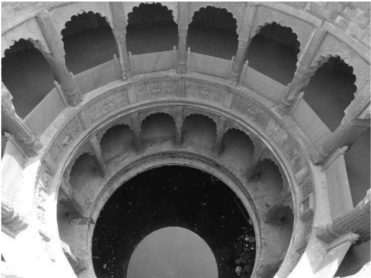
Dhaulpur-Chhoti Baodi-circular well shaft with galleries
