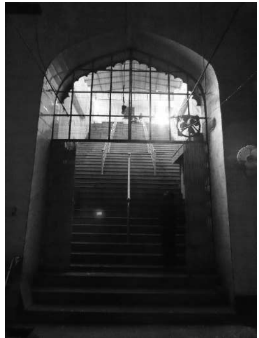
Shahpura-kali Mandir Baodi-view from the first tower towards the entrance
