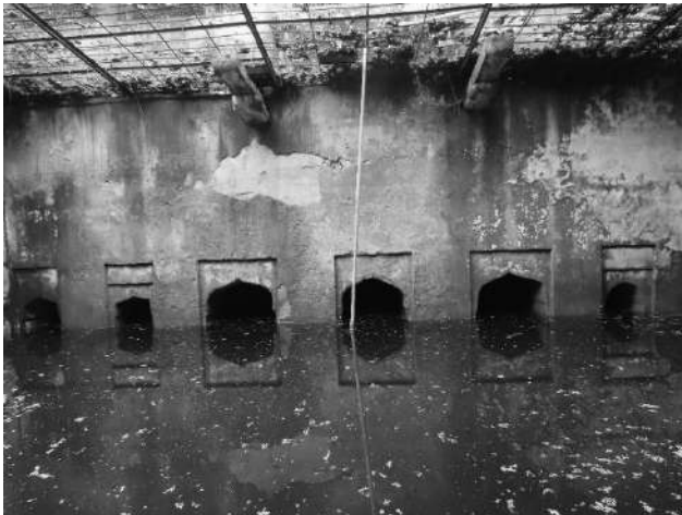
Kota-Abli Meeni Baodi-well shaft surrounded with corridors having openings towards well shaft
