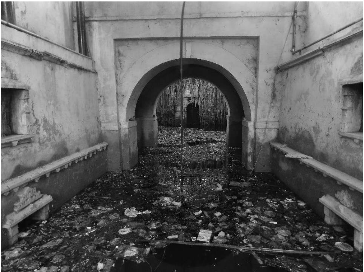
Udaipur- Sagasji Bavji temple baodi-view of the pavilion tower
