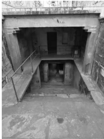
Sadri-Tarachand Kavedia Baodi- view while entering from north
