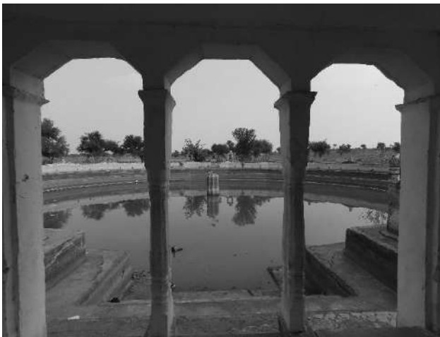
Untwaliya ka Johada-view through the openings of the entrance pavilion
