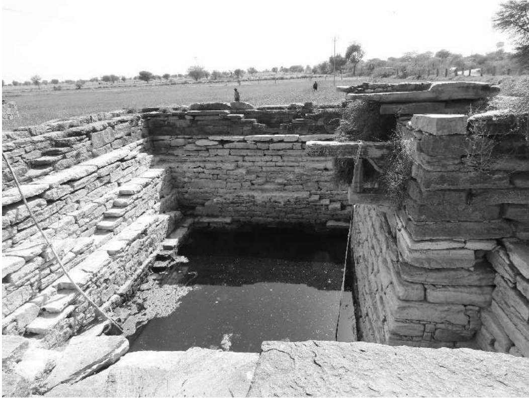
Moruda-Bhoot Baodi-looking towards south
