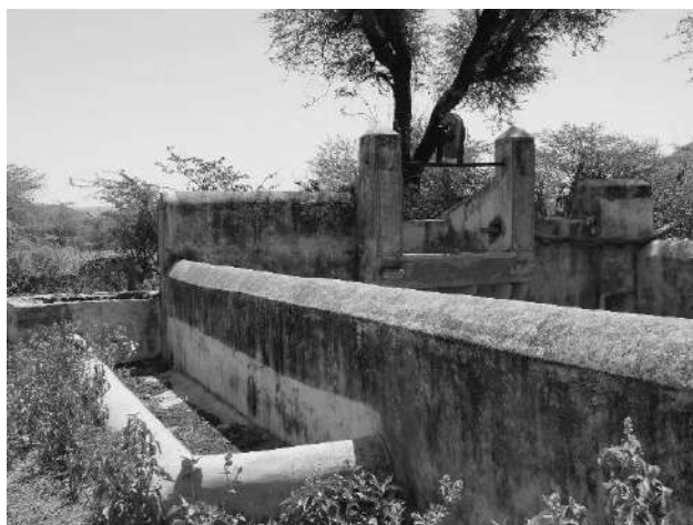
Tehla-Gopinath Mandir Baodi-trough for animals and water drawing arrangement
