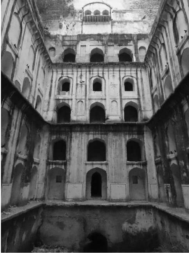
Jhujhunu-Meratni Baodi-third pavilion tower
