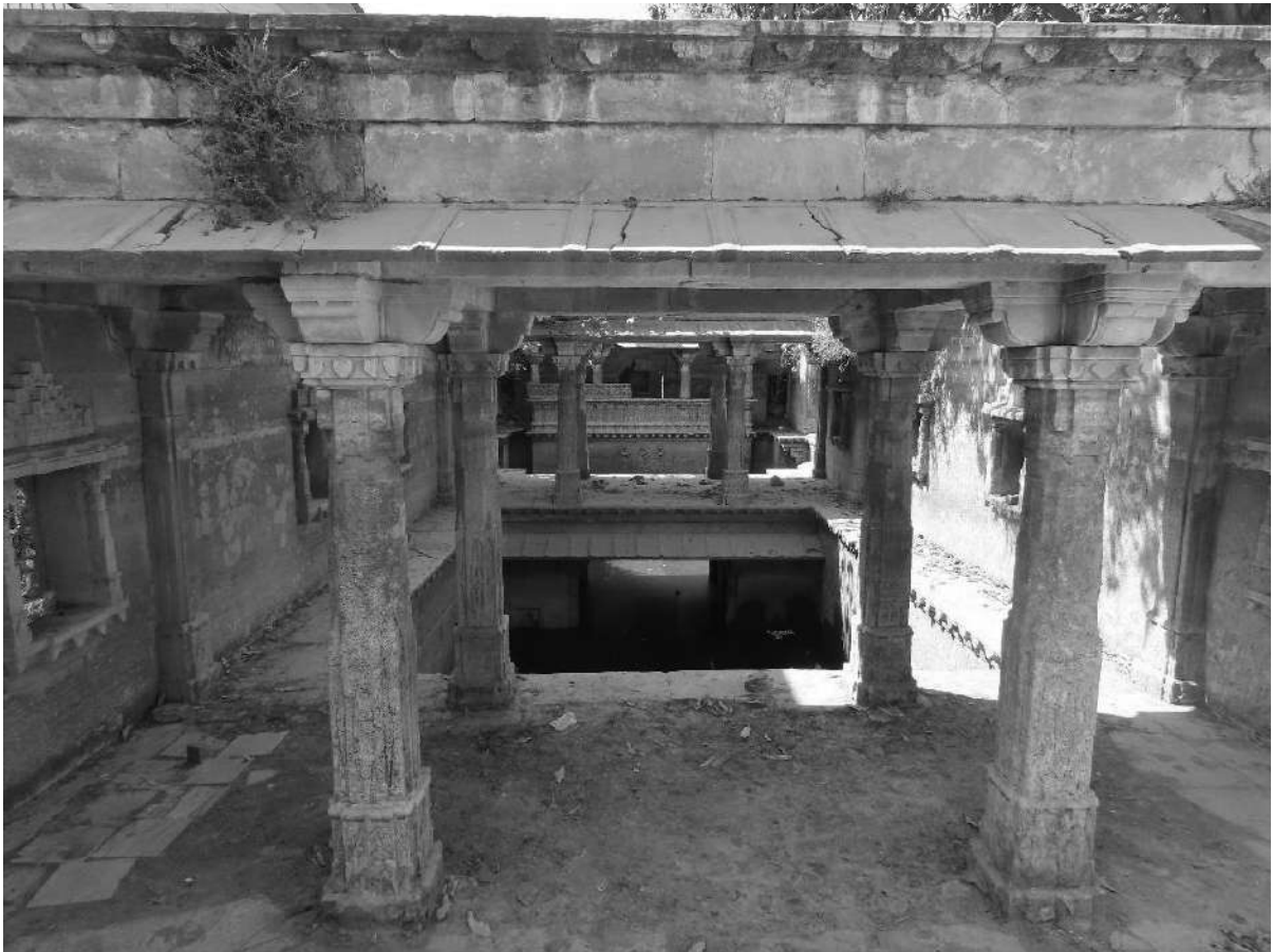
Udaipur-Trimukhi Baodi-view from the eastern entrance
