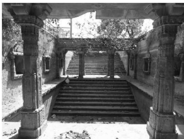
Udaipur-Trimukhi Baodi-view of the eastern entrance from the second pavilion tower
