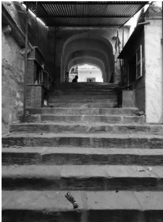
Ghanerao-Maili Vav-steps coming down from the road entrance through a series of arches
