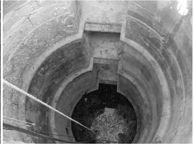
Sirohi-Baodi outside Sarneshwar Temple-well shaft with openings into the stepped corridor
