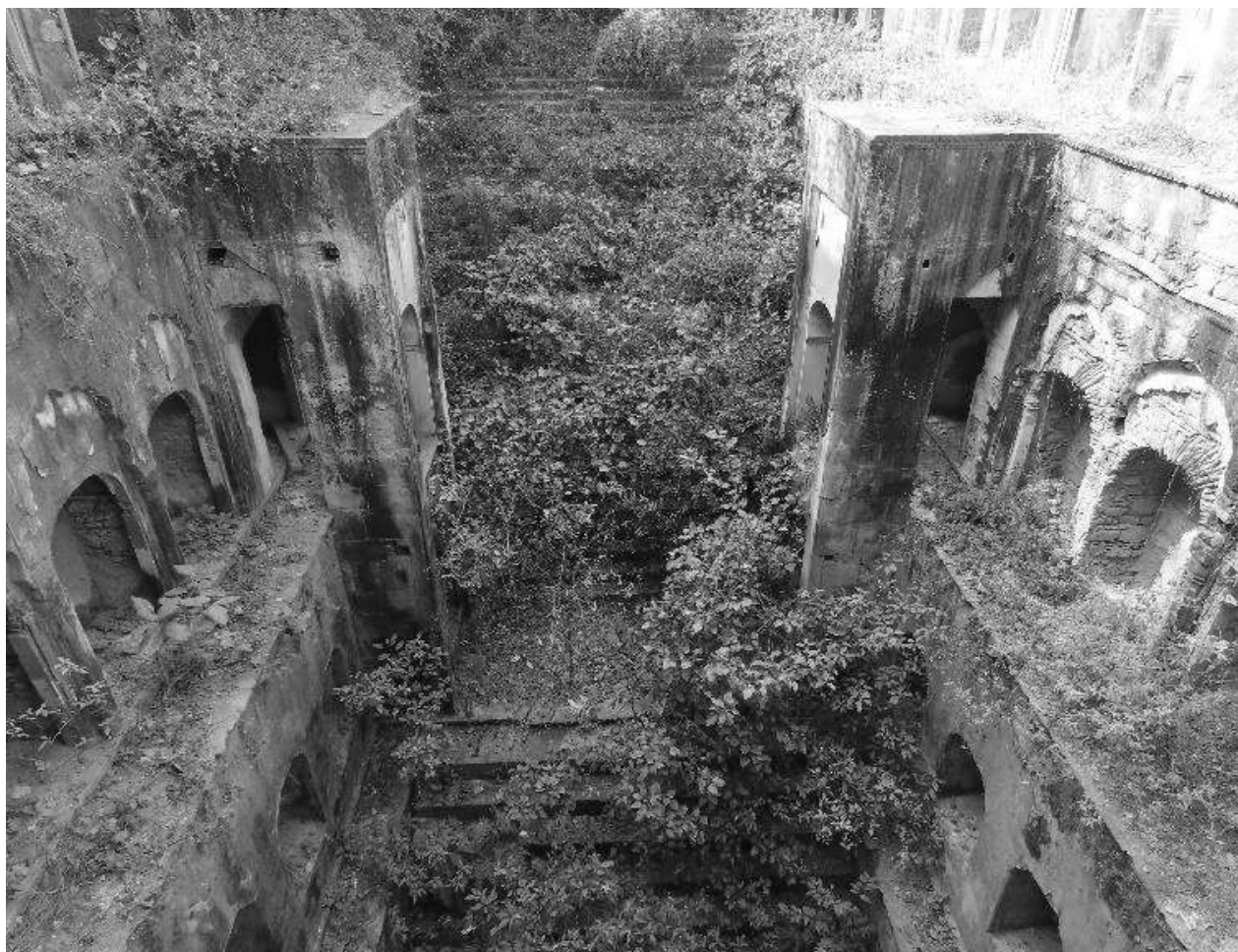
Rajgarh-Bheru Sahay ji ki Baodi-buttresses or counterfort supports at level 3 & 4
