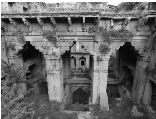
Khandela-Songiri Baodi-first pavilion tower when viewed from the entrance
