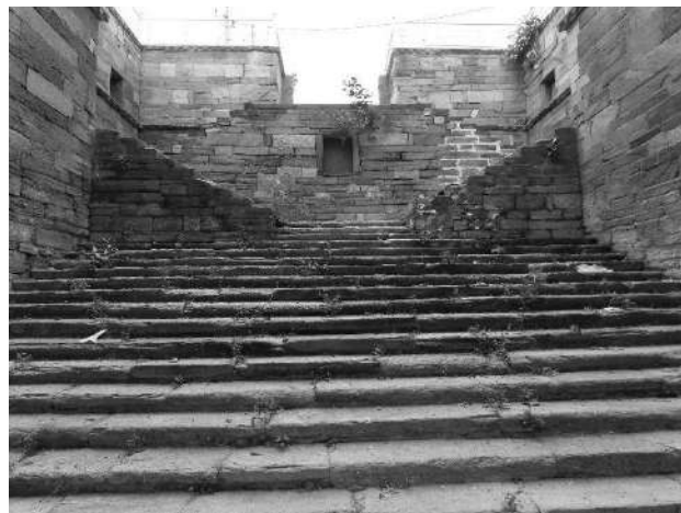
Toda Raisingh-Kingsi Baodi-view of the entrance in the east
