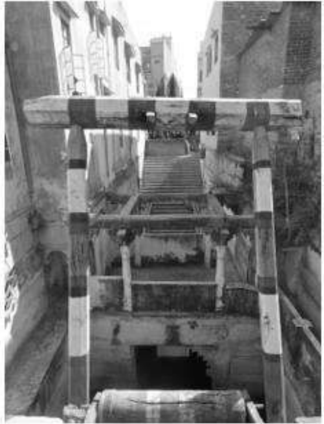
Bhinder-Hijron ki Baodi-view from the well shaft
