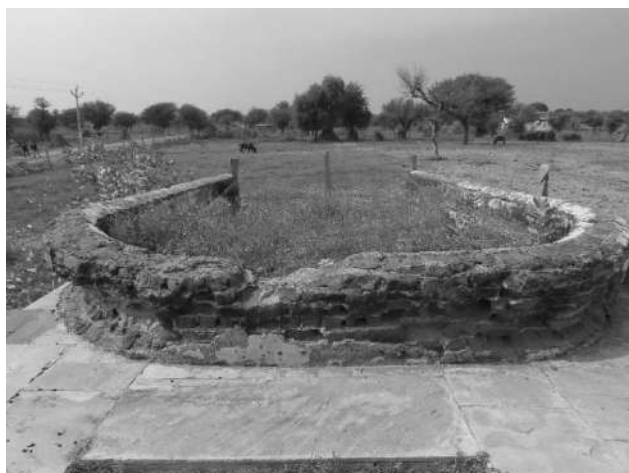
Lakshmangarh-Dholas ka Kua-track for bullocks for hauling up water
