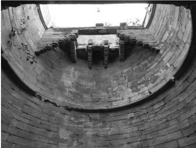
Balunda Stepwell-looking up the well shaft
