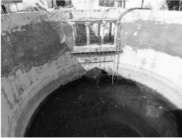
Merta City-Suwa Baodi-view from the east
