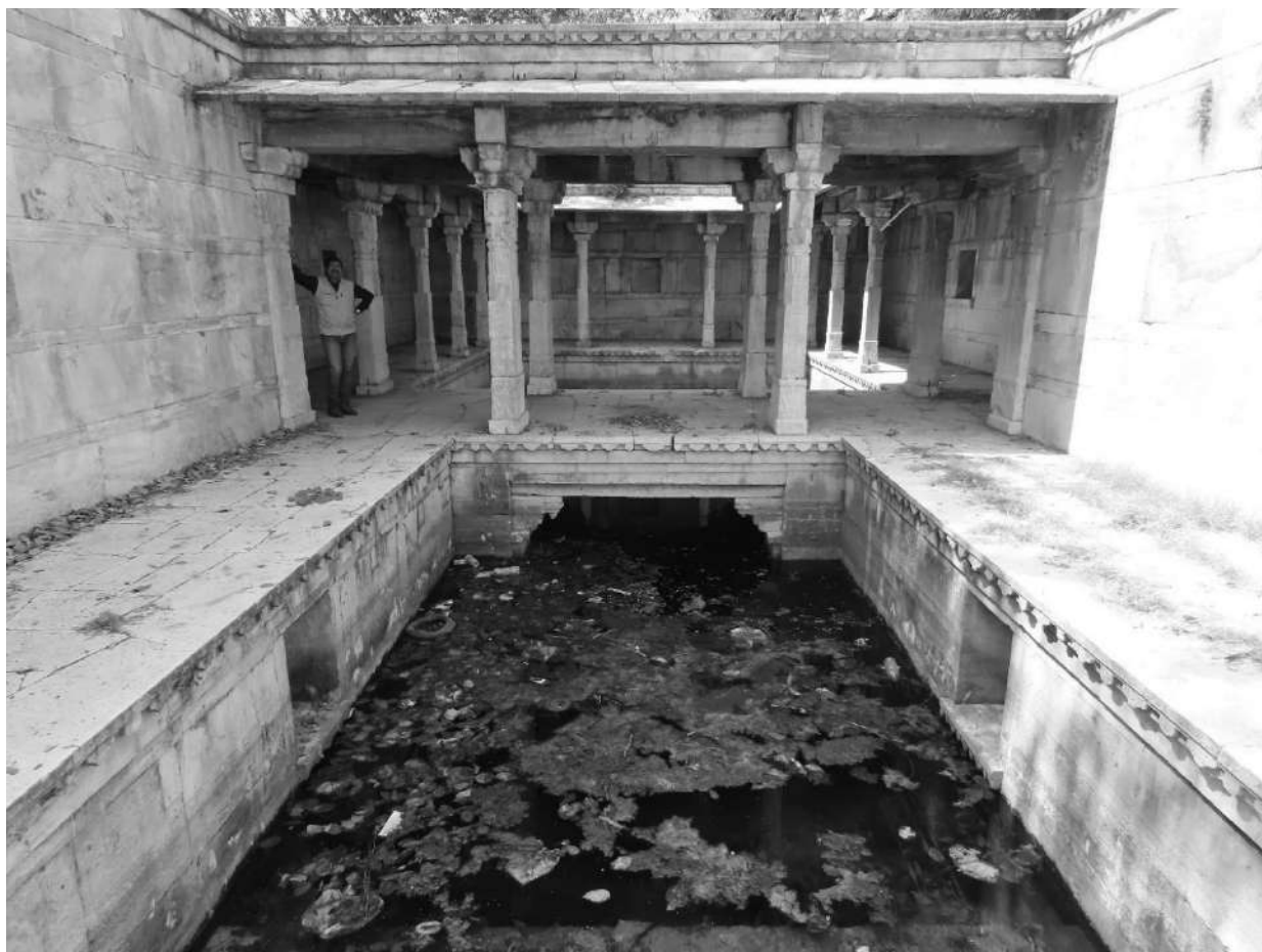
Udaipur-Bedla-Sultan Singh Baodi- view of the pavilion tower
