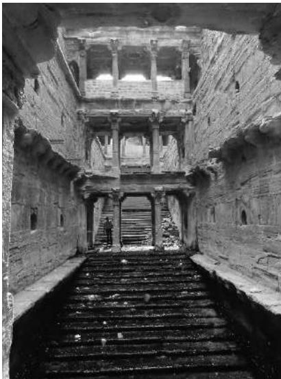
Jodhpur-Tapi Baodi- view of three storeyed pavilion tower, looking towards entrance
