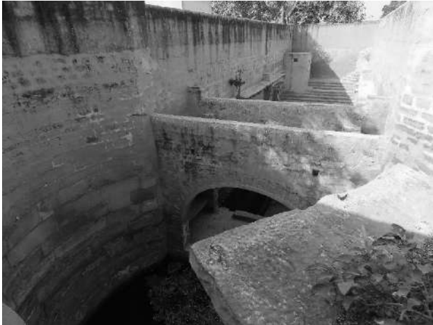
Merta City-Bum Baodi-view from the well shaft, restricted by walls erected all around the stepwell
