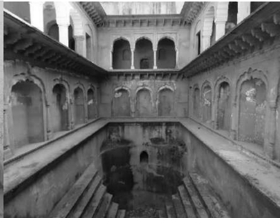
Shahpura Baodi-view of the second pavilion tower
