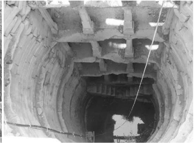
Nadol-Katwari stepwell-looking down the well shaft
